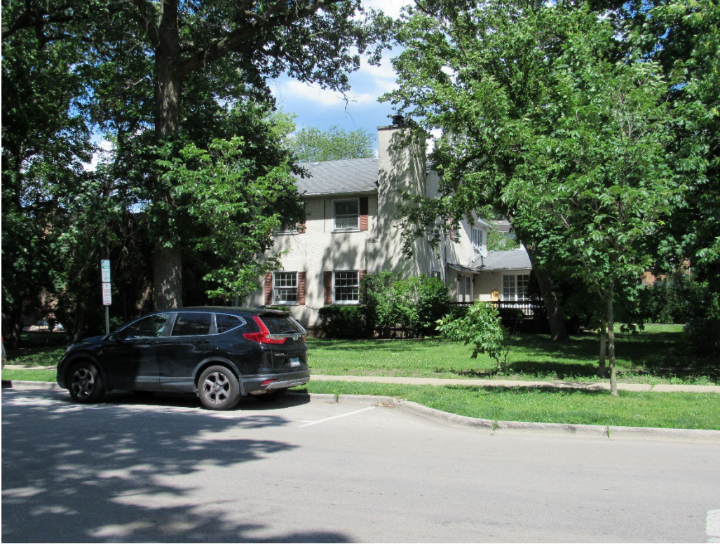
Photo 1 - Front Elevation (Linden Street)
