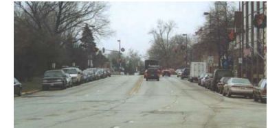
Unattractive streetscape with expansive cross-section Figure 64b
