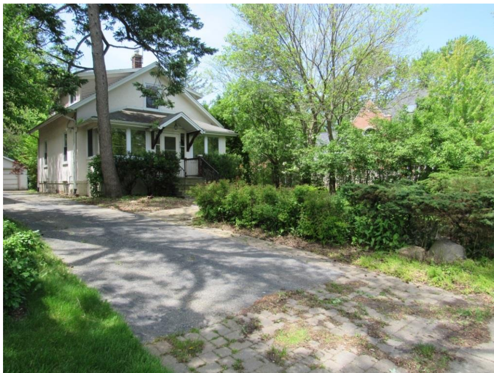
Figure 6 – Subject Property (688 Green Bay Road)
