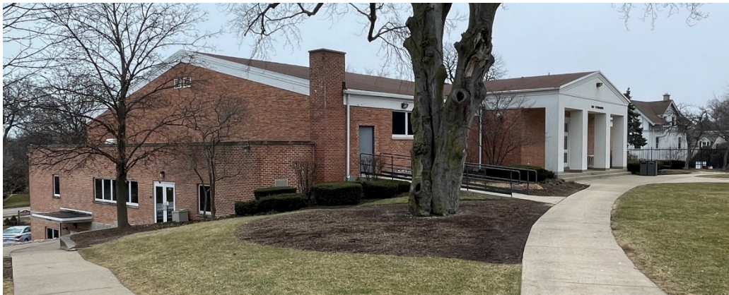
Figure 11 – Subject Property – Northwest façade of existing gymnasium
