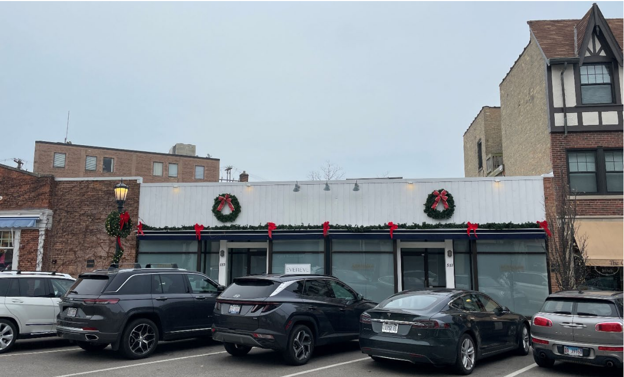
Figure 2 – Subject Property – Storefront facade along Chestnut Street
