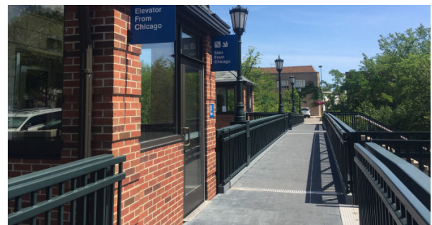
Access to elevators at Winnetka Metra Station.
