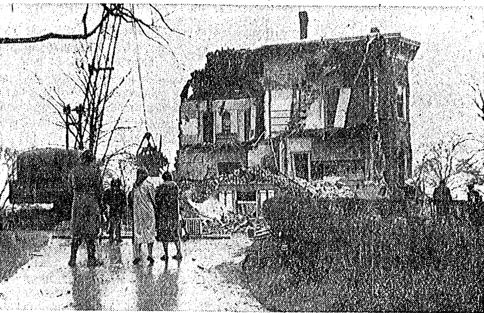
Knollslea hall, Winnetka, crumbles to ground. Building, once used for administrative offices of North Shore Country Day school, will be replaced by green lawn. John Garland Jr. built it in 1863.
