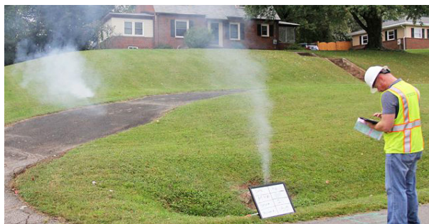
Smoke Testing © Pipe Spy
