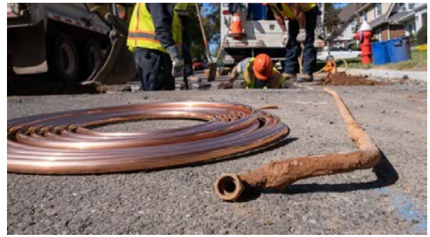
Replacing Lead Pipes © Chris Trento / Suez
