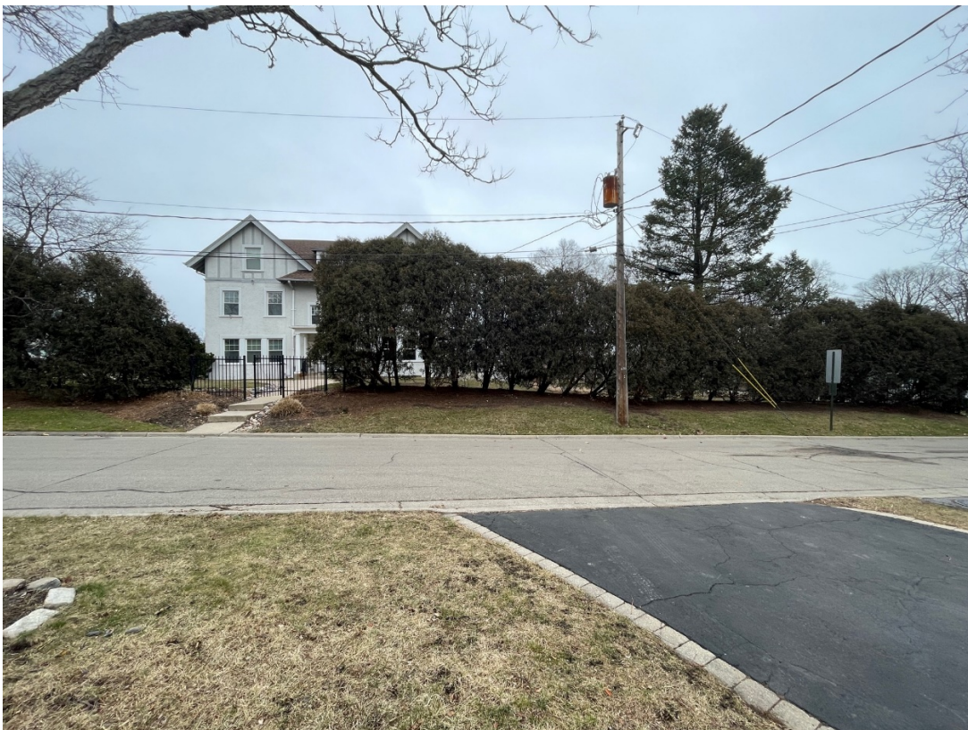
Figure 5 – Subject Property – South Elevation of Leicester Hall Looking From Elder Lane
