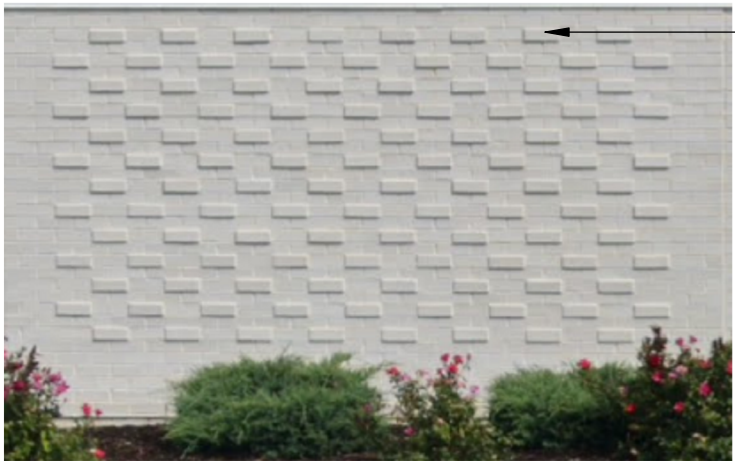
3 BRICK DETAILING - EXAMPLE OF PATTERN ONLY 1/8" = 1'-0"
