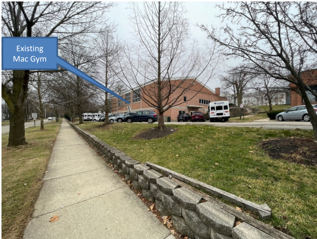
Figure 4 – Subject Property – North and East Elevations of Mac Gym Looking Southwest from Green Bay Road
