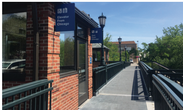
Access to elevators at Winnetka Metra Station.
