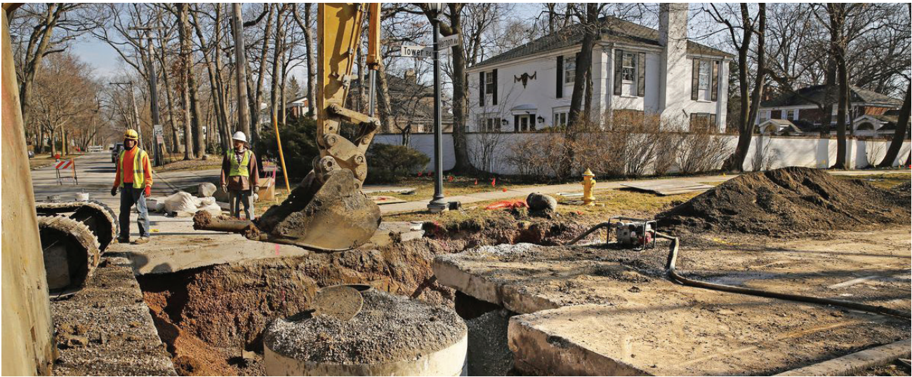
Storm sewer rehabilitation in Winnetka
