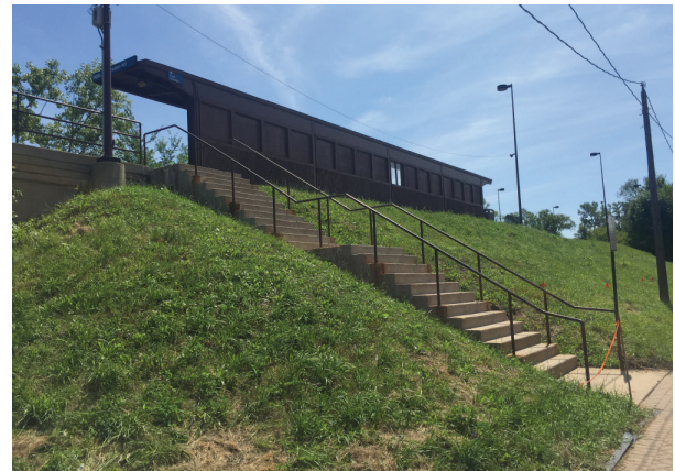
Stairs to Indian Hill Metra platform.
