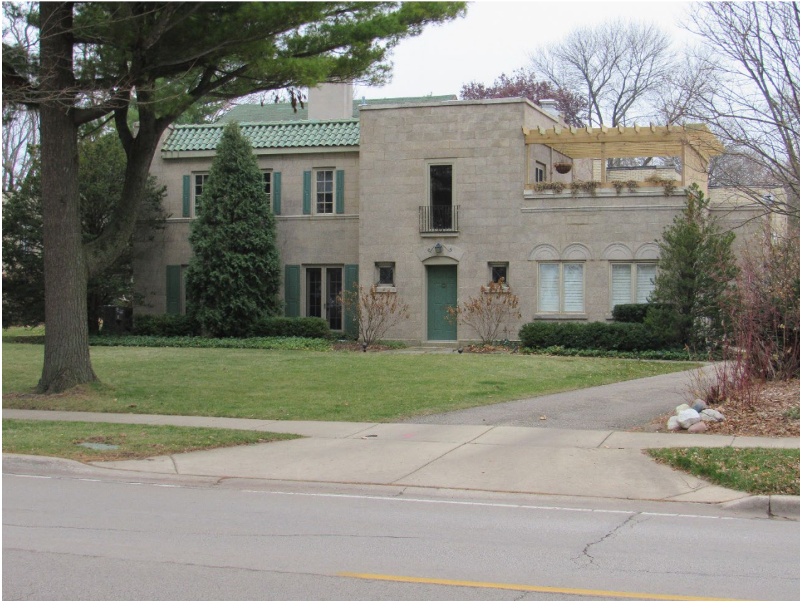
Figure 4 – Subject Property (Front Elevation – Sheridan Road)
