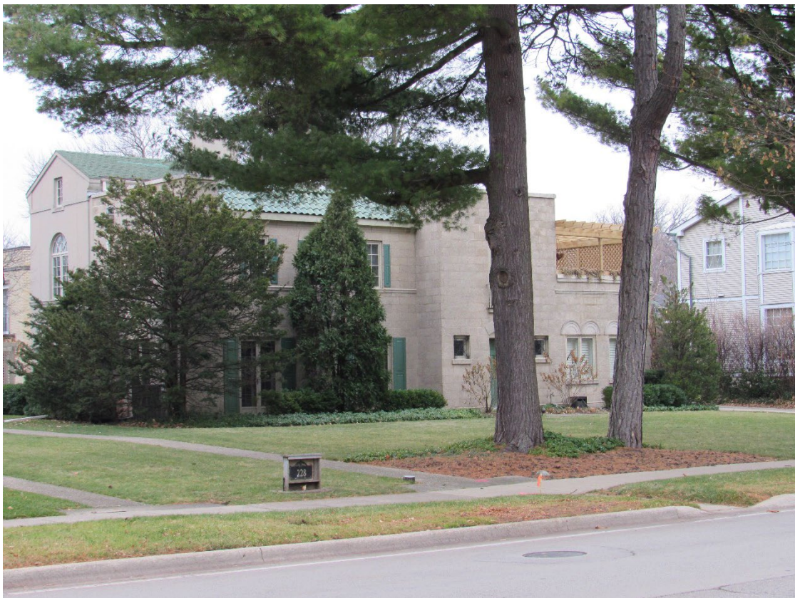
Figure 5 – Subject Property (Southerly Front Elevation)
