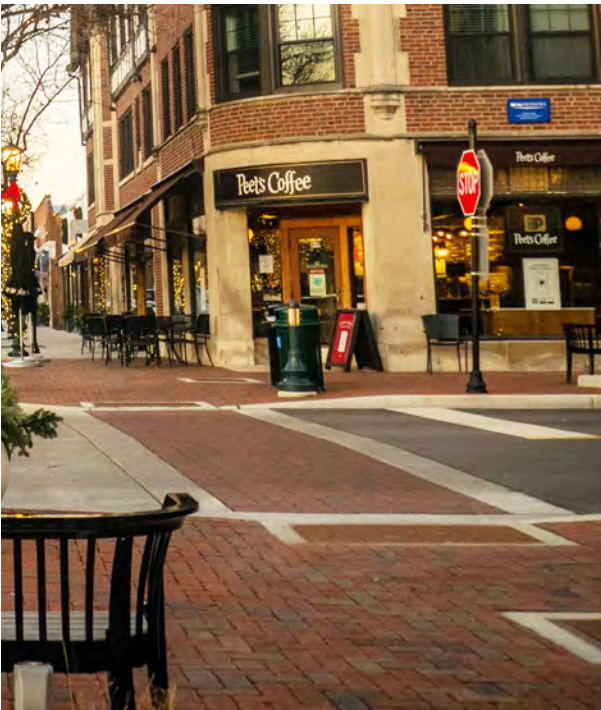
Accessible Curb Ramp - West Elm © Village of Winnetka
