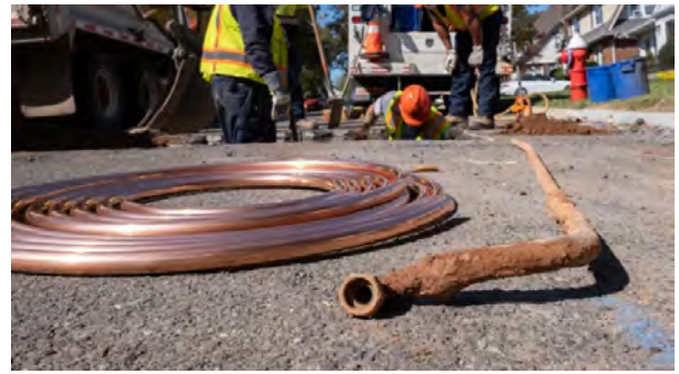
Replacing Lead Pipes © Chris Trento / Suez
