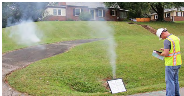
Smoke Testing © Pipe Spy
