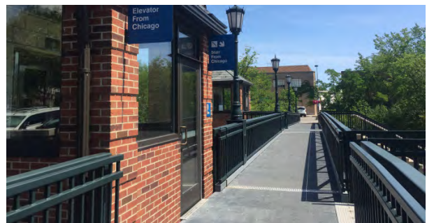
Access to elevators at Winnetka Metra Station.
