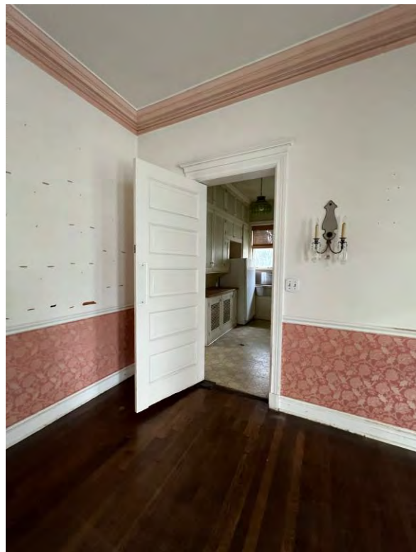
Dining room north wall, view to kitchen
