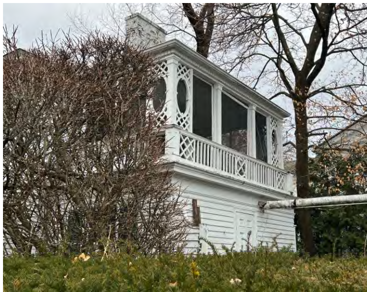
East façade of garage
