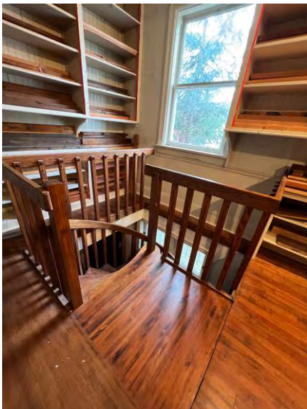
Pantry looking northwest
