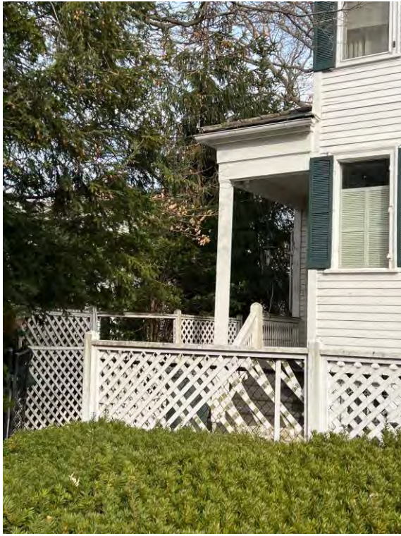
West façade, north service entrance
