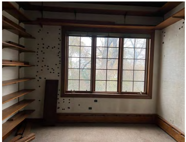
Enclosed south porch, east wall
