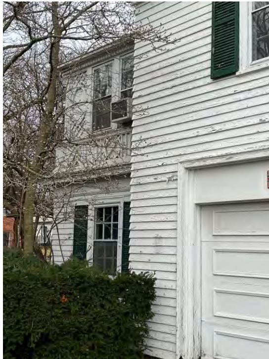
South façade, west end of garage
