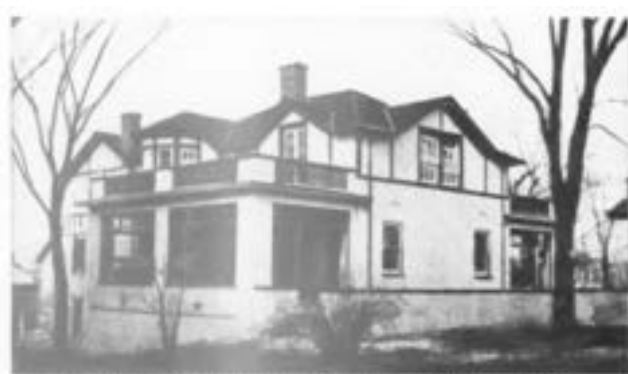
The Home of A. J. Hardy, Evanston. William A. Otis and Edwin H. Clark, Architects
