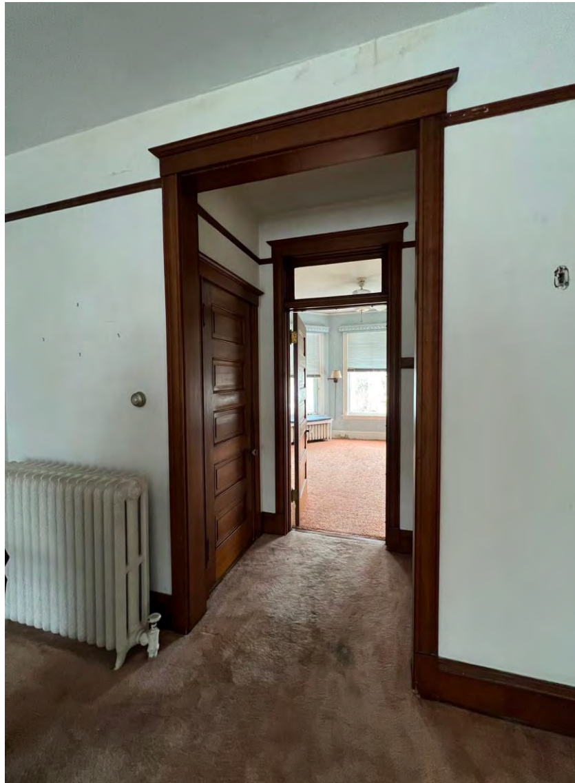
Hall looking east into east bedroom
