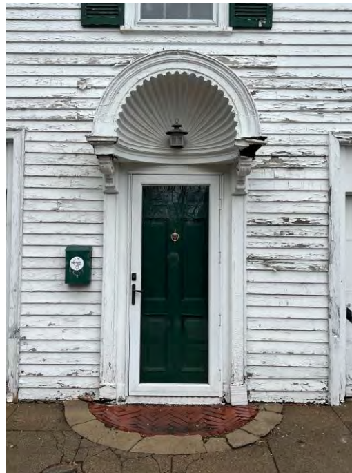
Garage, south façade and front entry
