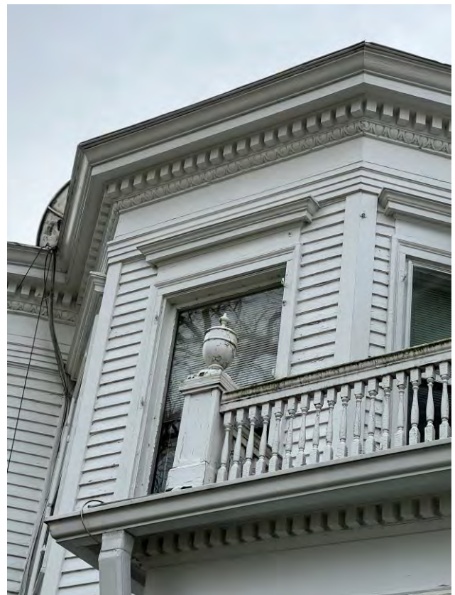
East façade second floor porch
