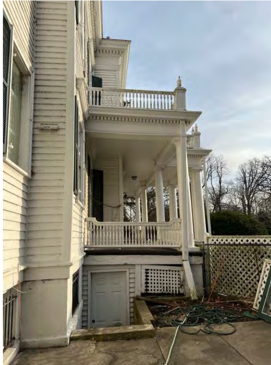
North façade of front porch
