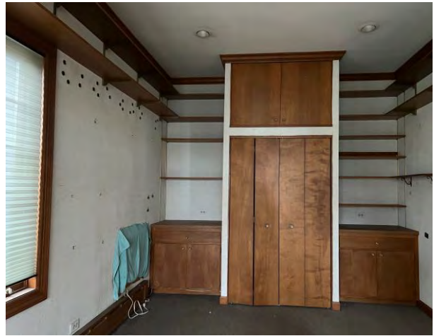
Enclosed south porch, west wall
