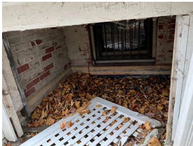
North façade, foundation
