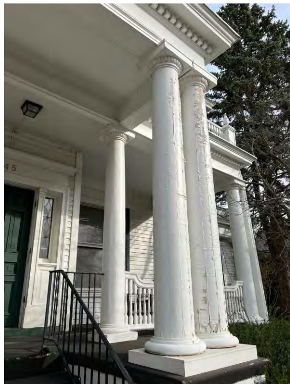
West façade details
