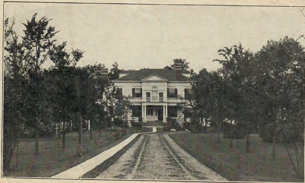
Residence of Everett Wilson, Winnetka, Ill., Sheridan Road near Pine Street.
