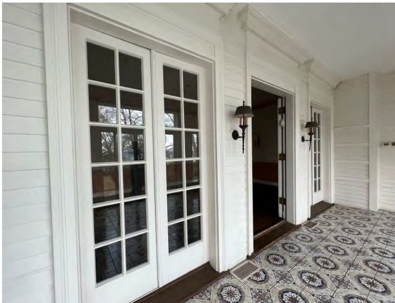
Enclosed east porch looking northwest
