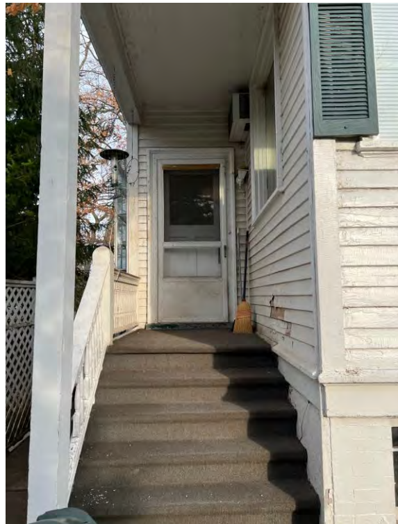
West façade, north service entrance
