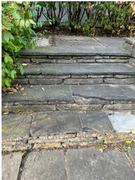
South terrace stairs to south garden
