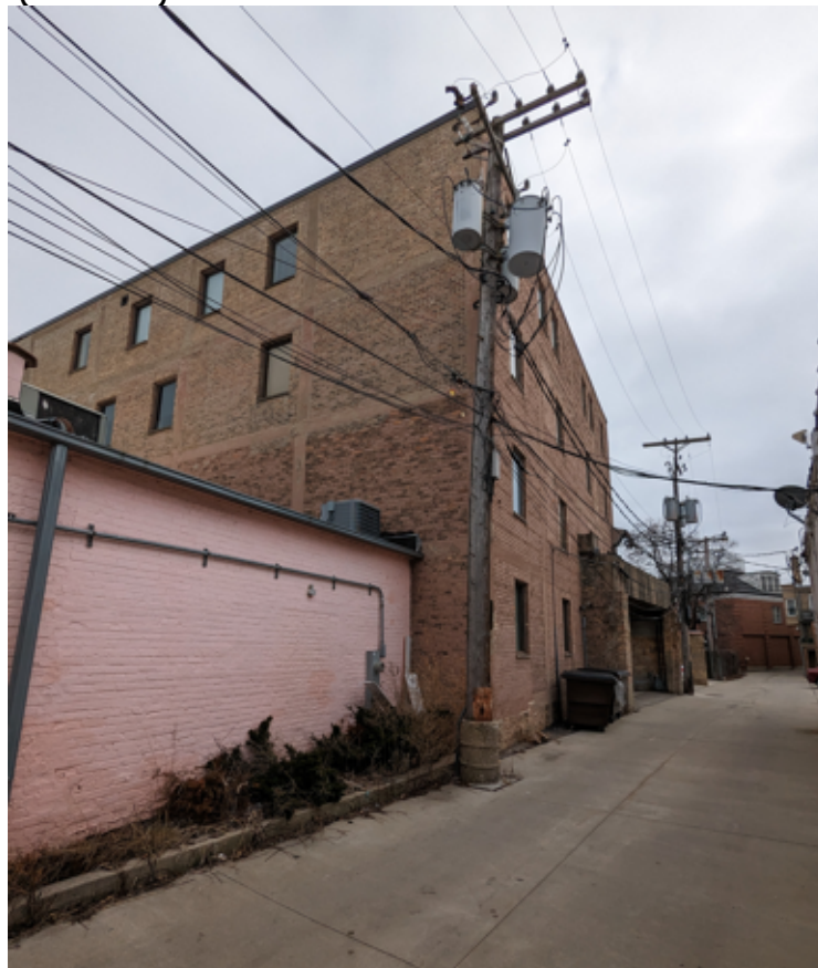
Adjacent Buildings on Green Bay Rd
