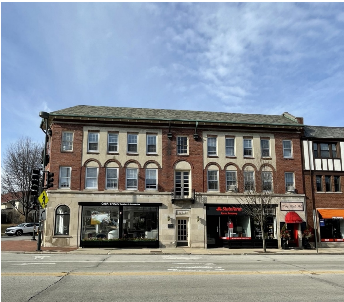
Figure 2 – Subject Property – East Façade/View from Green Bay Road
