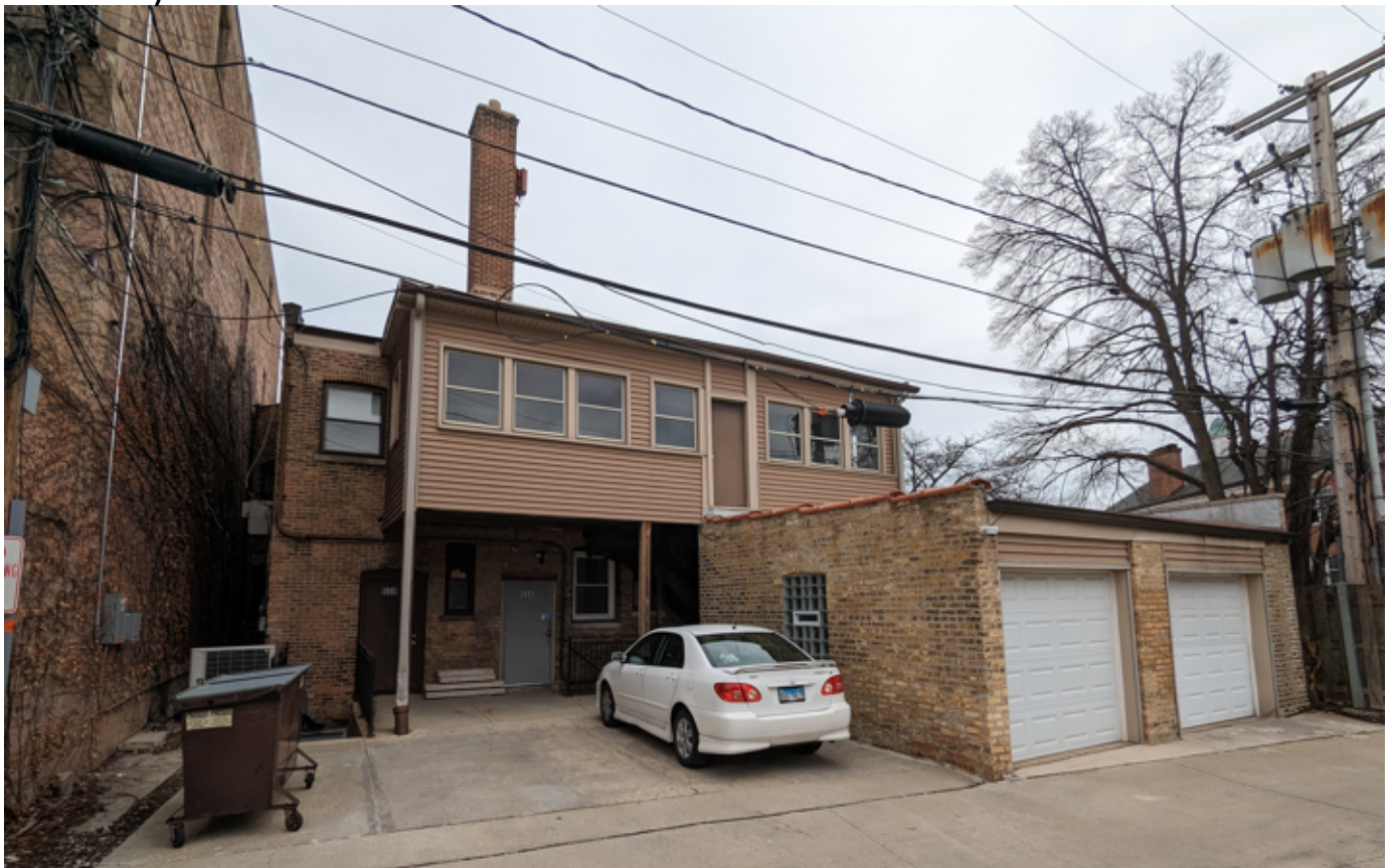
Adjacent Buildings on Green Bay Rd
