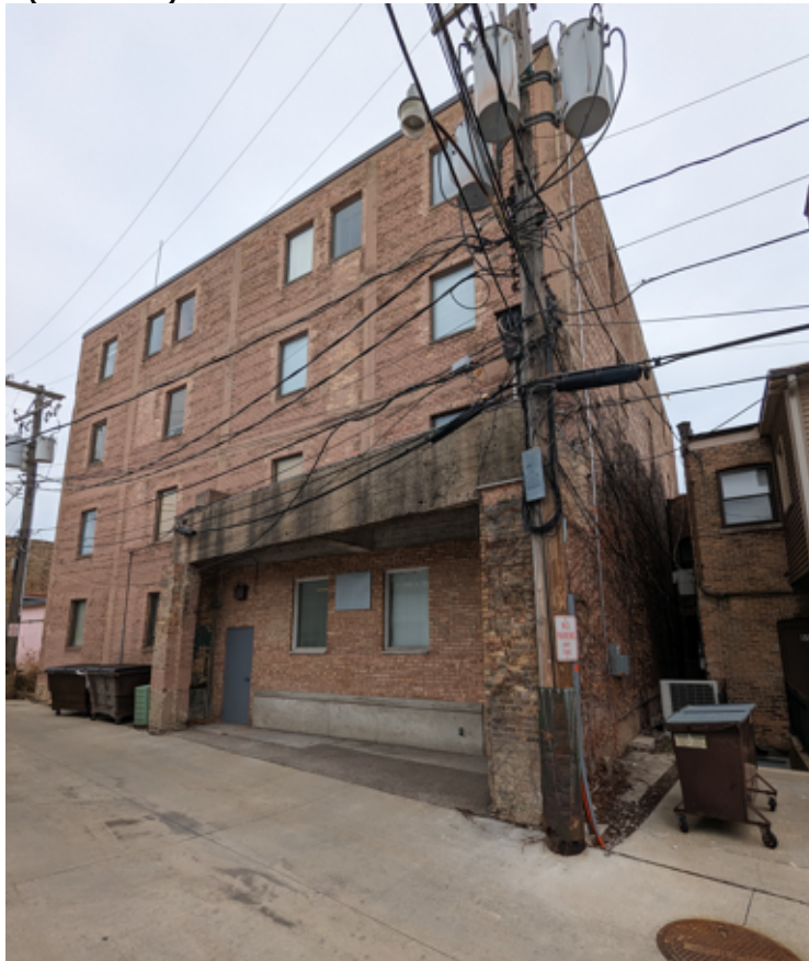
Alley at 560 (south)
