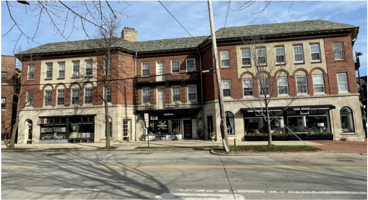
Figure 1 – Subject Property – South Façade/View from Tower Road
