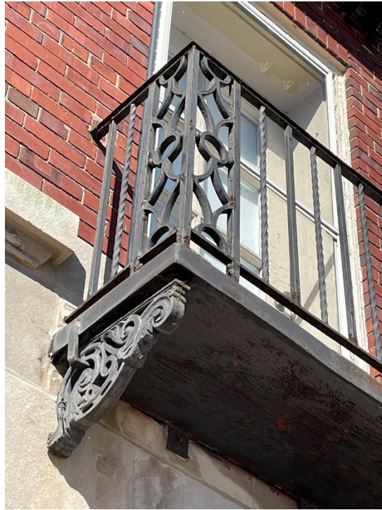
Figure 3 –Typical existing balcony iron guardrail detail
