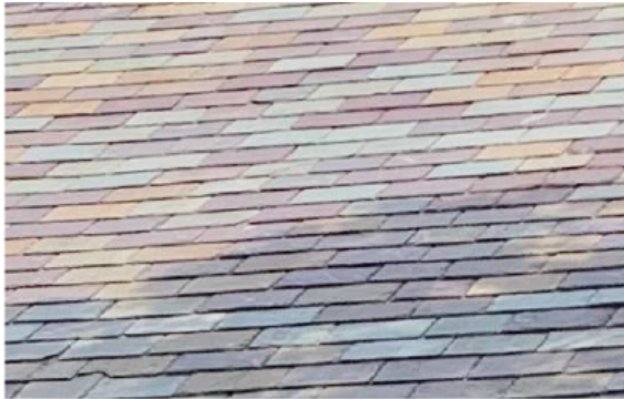
NEW SLATE ROOF TILE, TO MATCH EXISTING
