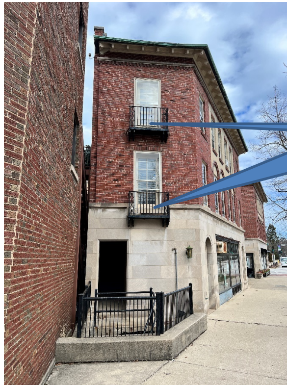
Figure 6 – Subject Property – West building façade
