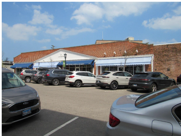
555-571 Chestnut Street (commercial building to west)
