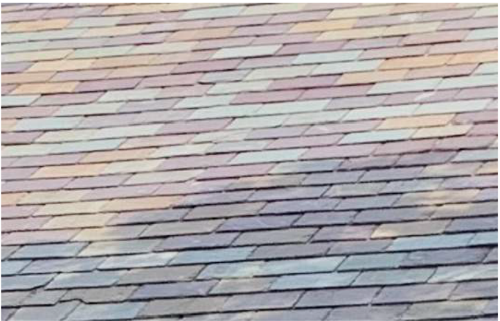
NEW SLATE ROOF TILE, TO MATCH EXISTING
