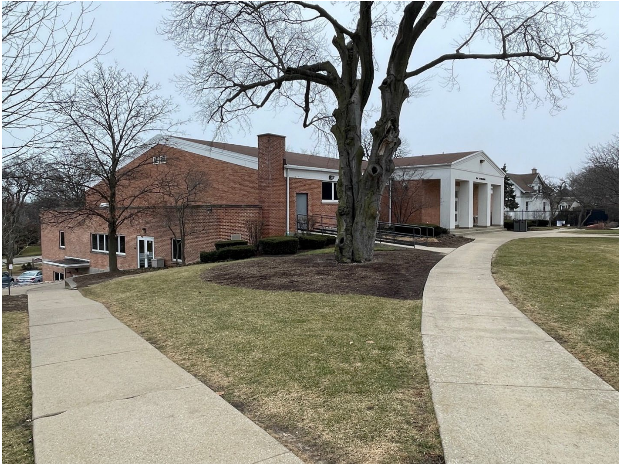
Figure 6 – Existing Mac Gym – North and West Elevations Looking from Interior Campus to the Southeast
