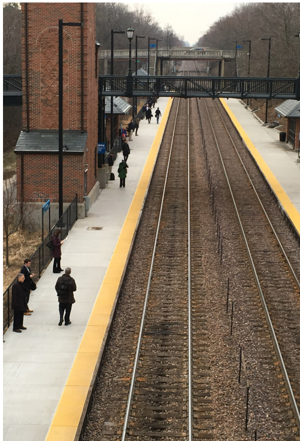
Metra UPN Train Tracks
