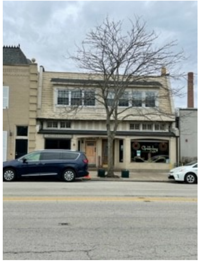
566-568 Green Bay Road (mixed-use building to north)
