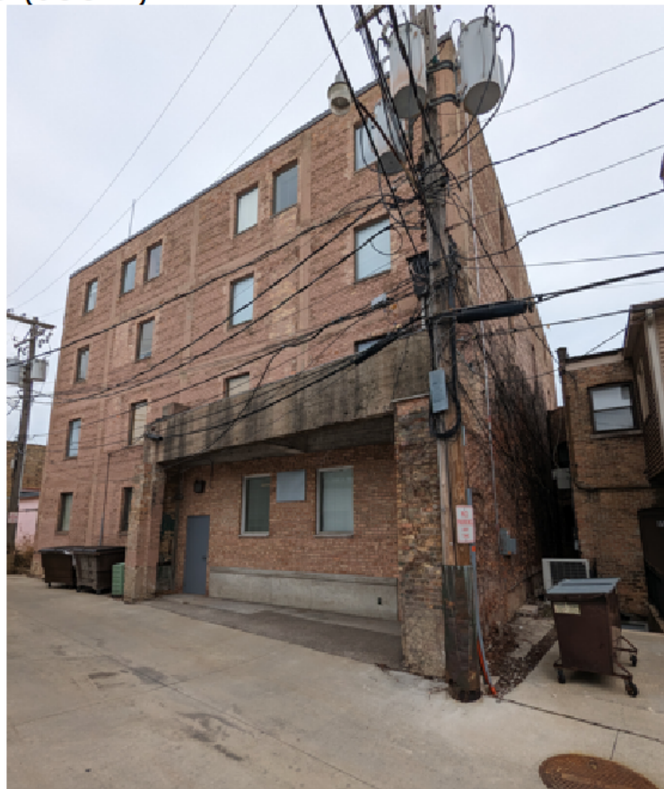
Alley at 560 (south)
