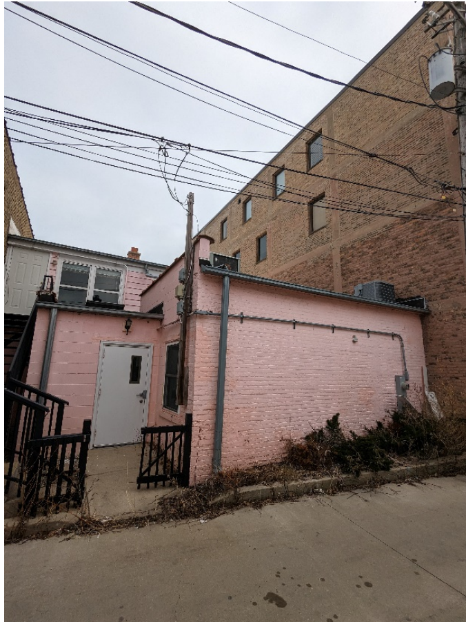
Figure 3 – Subject Property – Existing Rear Building Elevation
