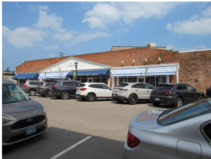
555-571 Chestnut Street (commercial building to west)
