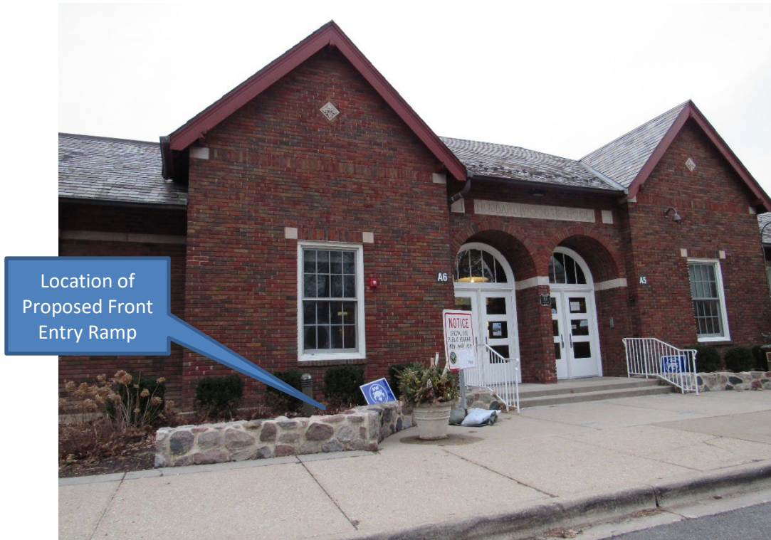
Figure 5 – Subject Property – Front Elevation (Chatfield Road) – Looking South
