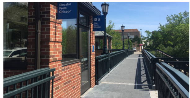
Access to elevators at Winnetka Metra Station.
