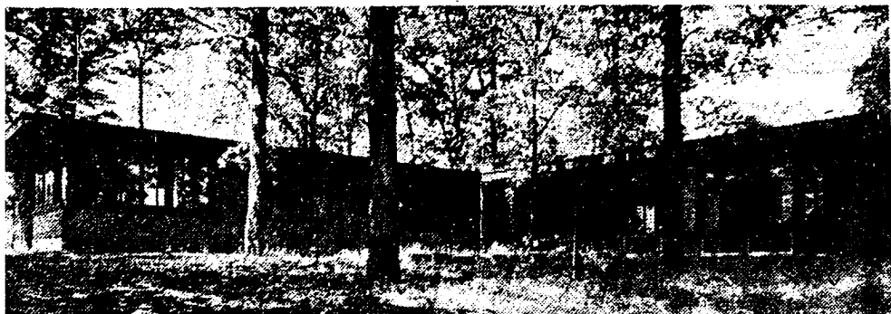
The Marvin Fitch home on Osage st., Park Forest, built on wooded lot, is of common brick and redwood, with large windows. View is from the rear.
