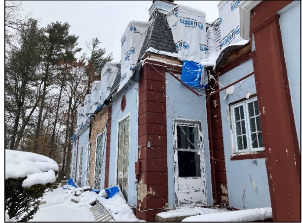
Rear (west) façade looking north
