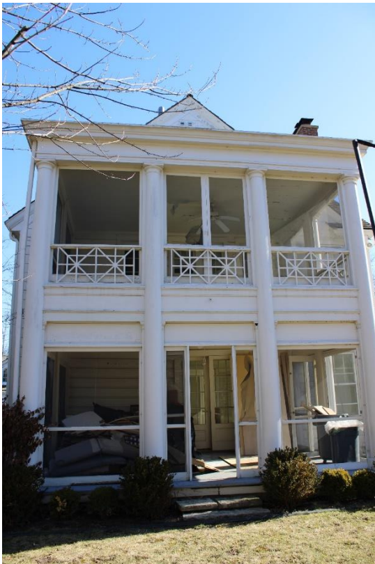
West façade, view east.
