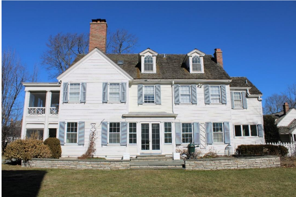
South façade, view north.
