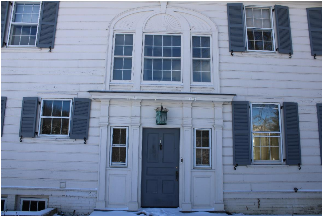
Front entrance detail.
