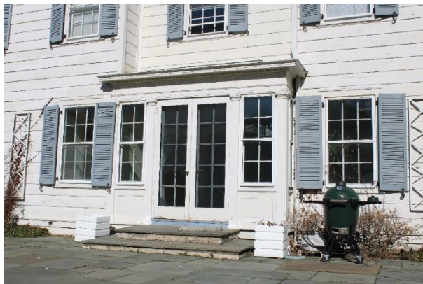
South façade entrance.
