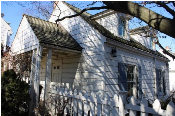
South garage, view northwest.
