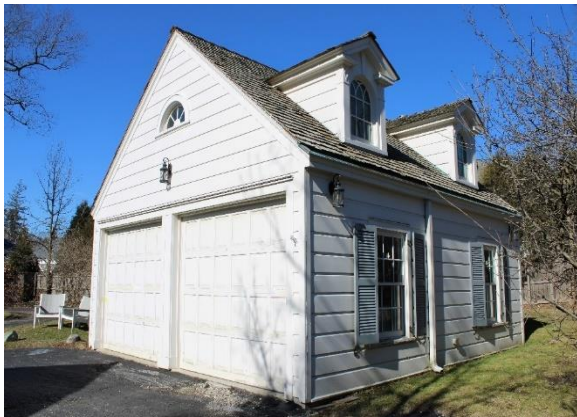
North garage, view northwest.
