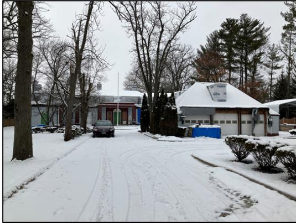
Front (east) façade looking west
