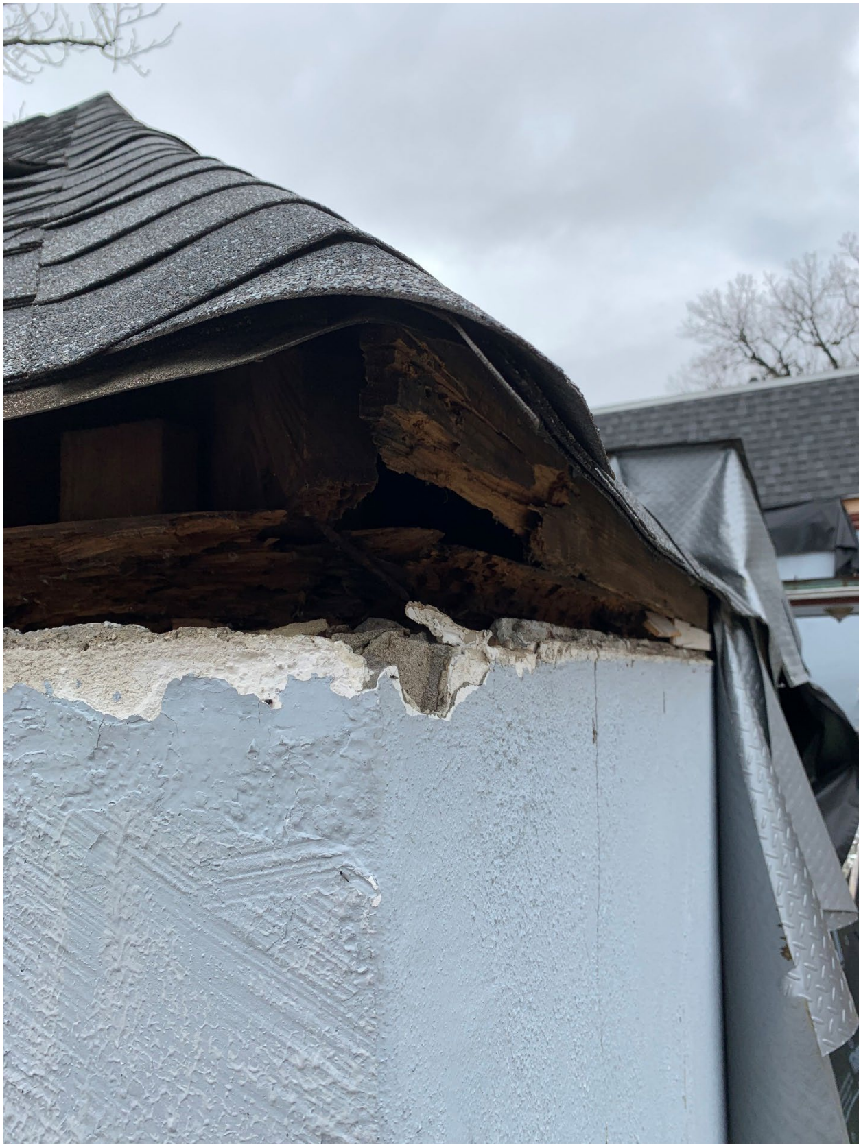
Figure 11 - close up of garage wall / roof intersection
