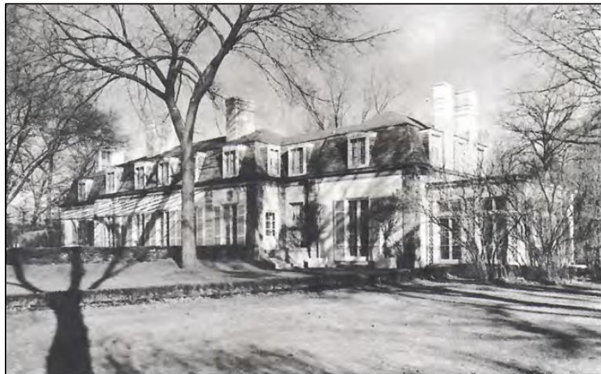
West façade and terrace, 1950
