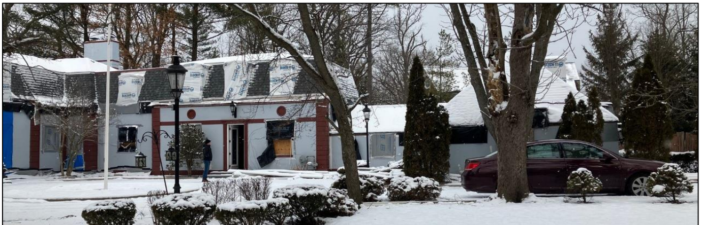
Looking north at the front (south) façade of the service wing and garage.
