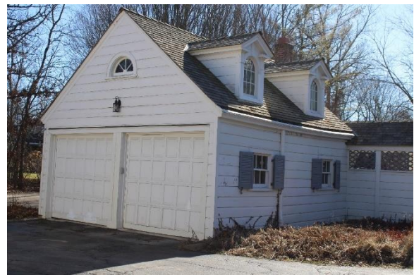
South garage, view southeast.
