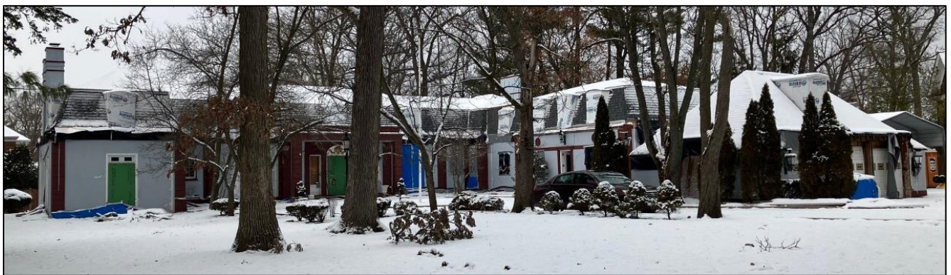
Front of house, looking northwest.
