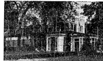
View of the Maremonts' Versailles manor house, taken from the broad lawns which give it its name, Tapis Vert.
