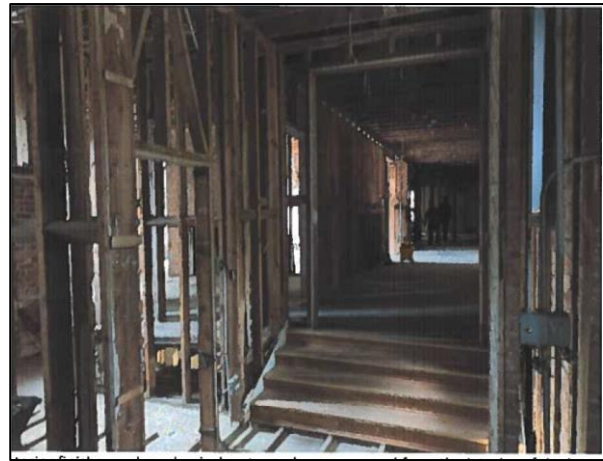
Looking N to main hall from living room
