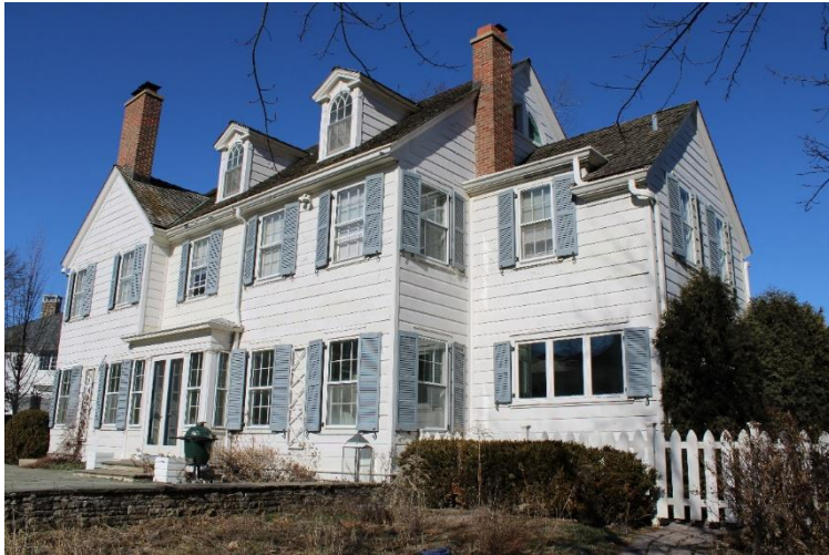
Rear (south) façade, view northwest.
