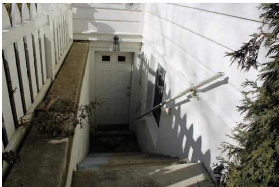
Basement door, east façade.
