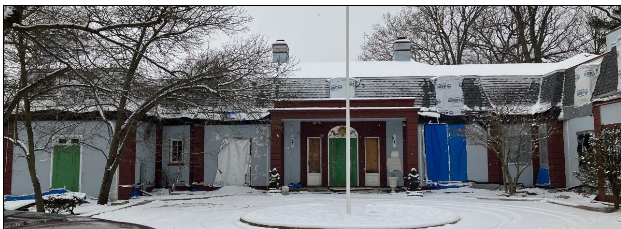
Front (west) façade of main house, looking west.
