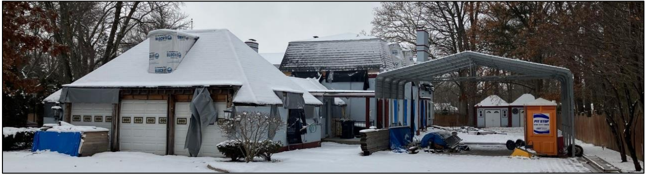
Looking southwest at the garage and the east end of the north façade.
