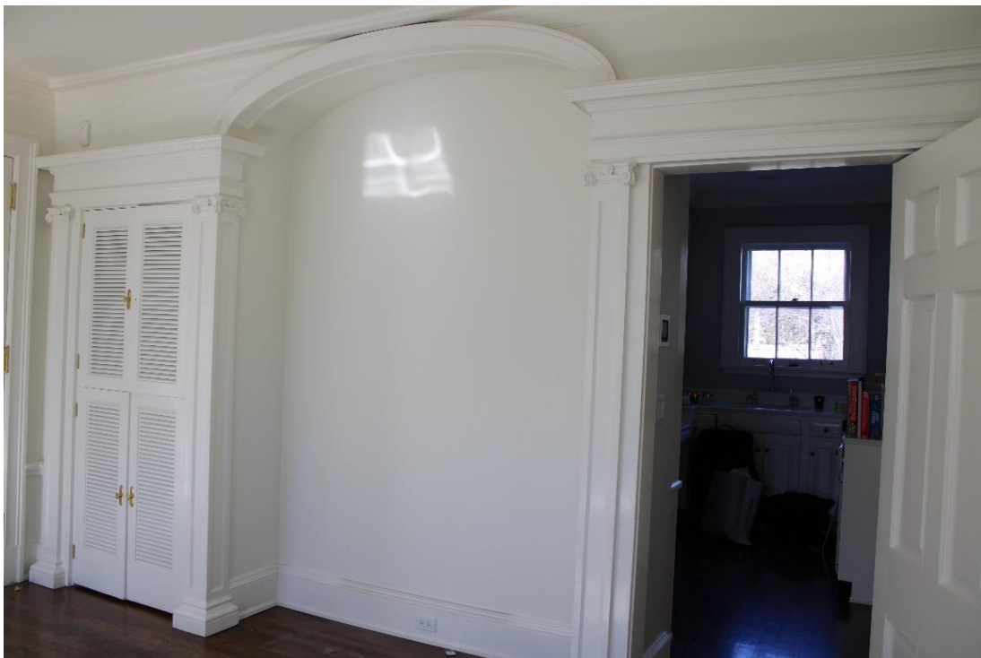
Dining Room alcove with Classical detailing.
