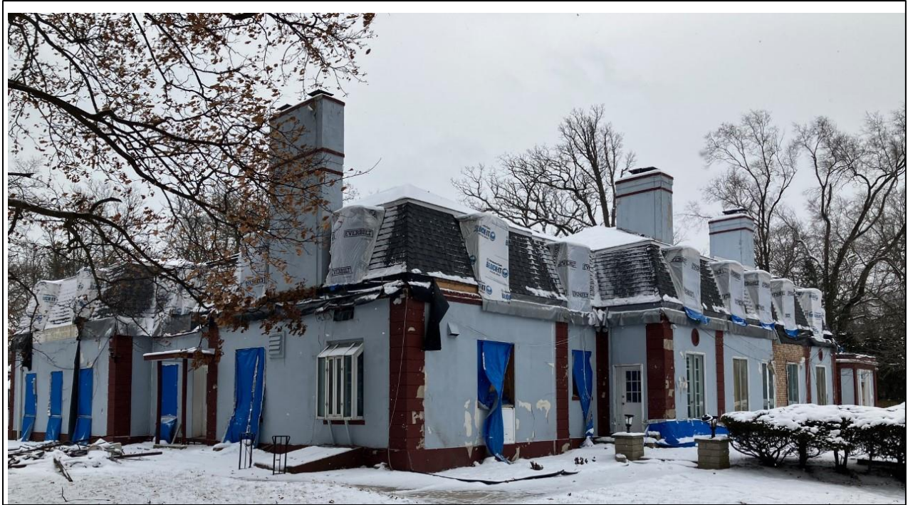
Looking southeast at the rear (west) and the rear third of the side (north) facades.
