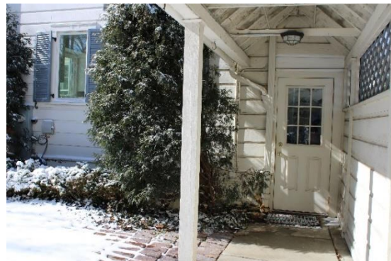
Side door, east façade.
