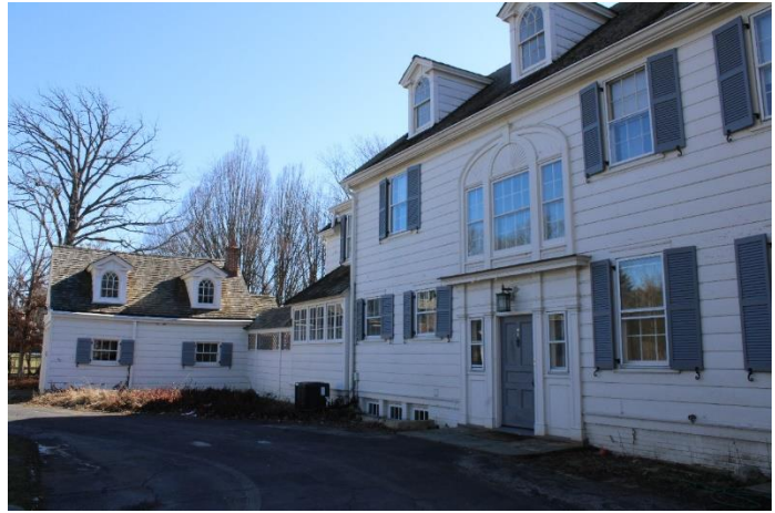
Front façade, view east toward south garage.
