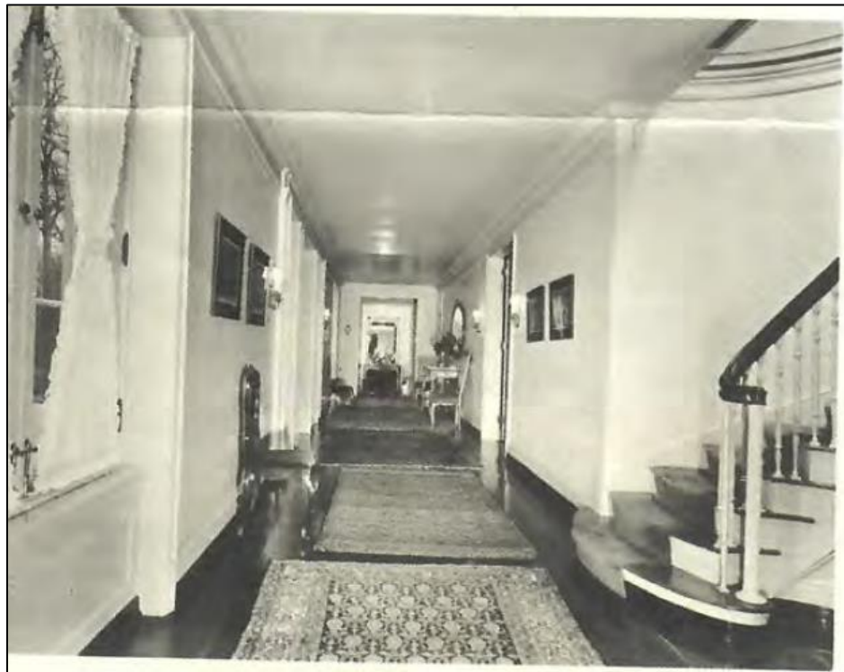
1 st floor hall of main house, looking south from main staircase, 1950
