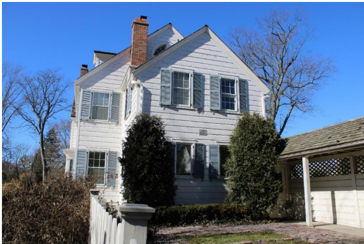
East façade, view west.
