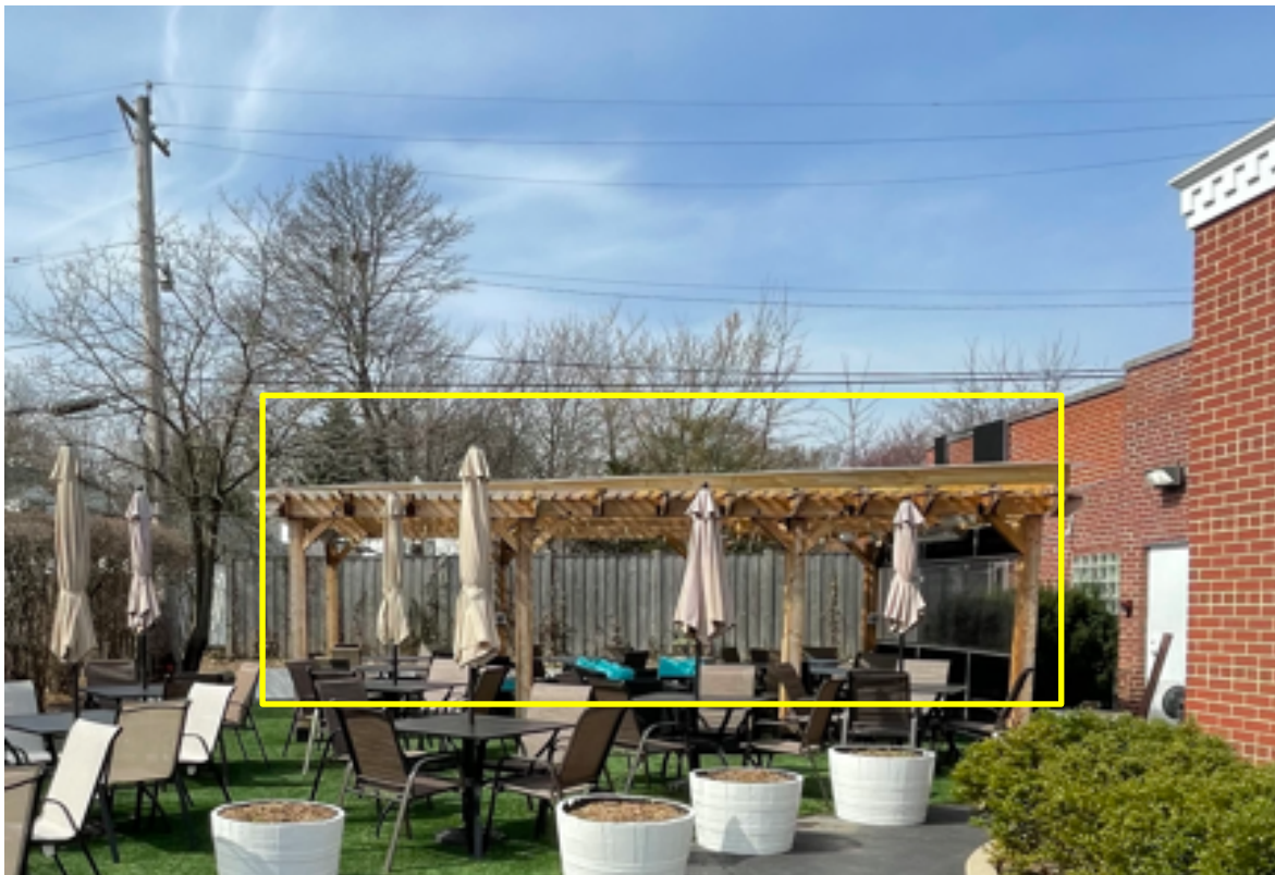
Figure 2 – Subject Property – West Façade/Existing pergola/View from the Green Bay Road
