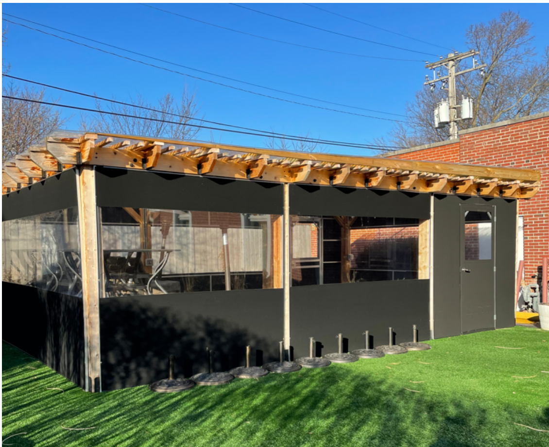
Figure 4 –The closer look at the existing pergola (with side panels)/ West Façade
