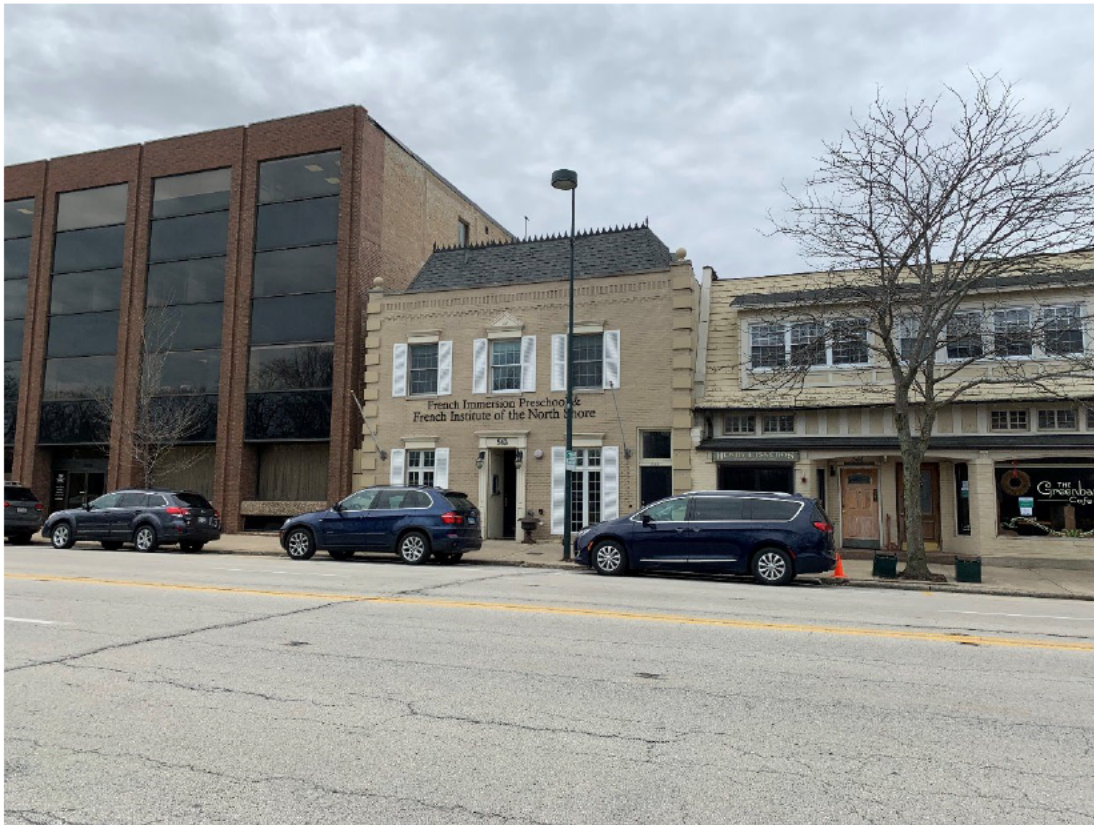
Figure 3 – Subject Property with Neighboring Properties
