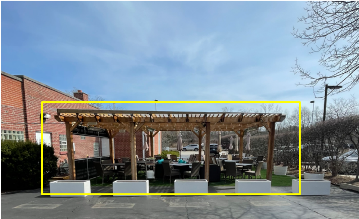
Figure 3 – Subject Property – South Façade/Existing pergola view from the Green Bay Road alley
