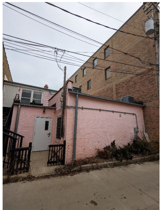
Subject Property – Rear Building Elevation (Alley)
