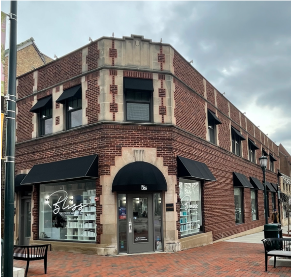
Figure 1 – Subject Property – Chestnut and Elm Street intersection, north and west facades (April 2023)
