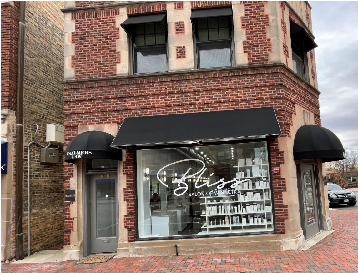
Figure 2 – Subject Property – North façade along Elm Street (April 2023)
