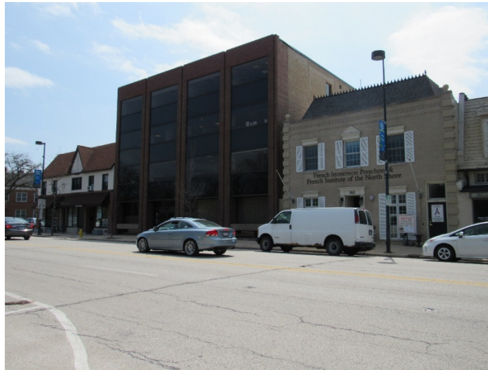
Subject Property with Neighboring Properties to South
