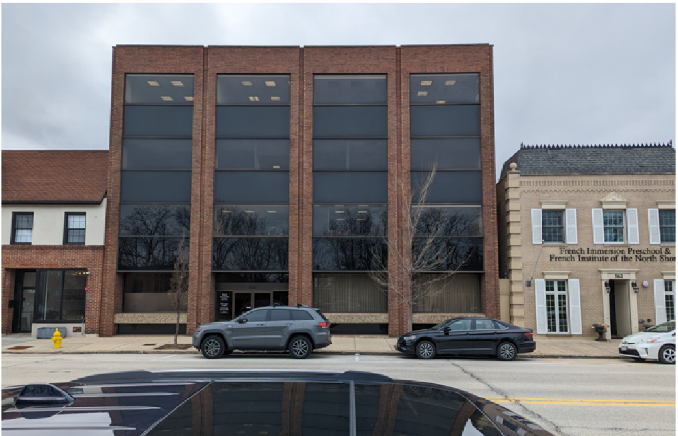
Adjacent Buildings on Green Bay Rd to South
