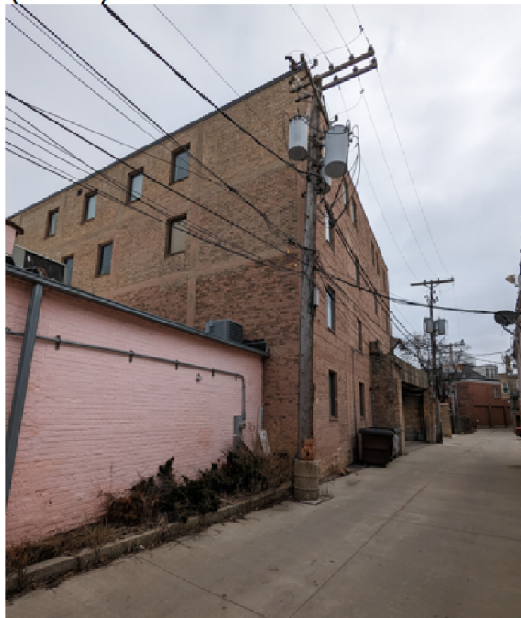
Adjacent Buildings on Green Bay Rd
