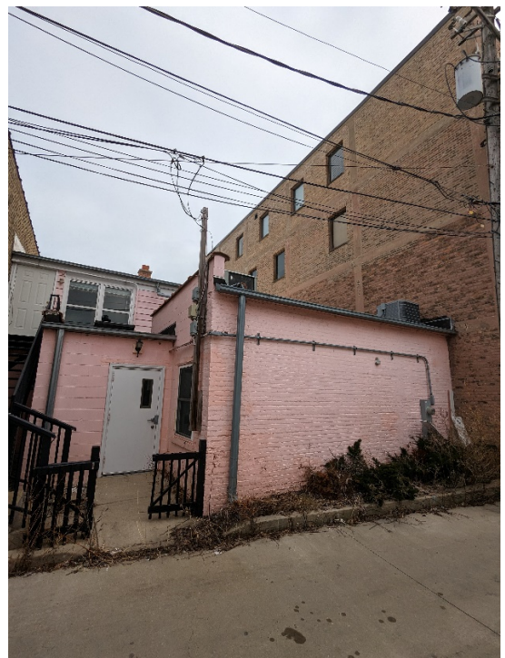
Subject Property – Rear Building Elevation (Alley)
