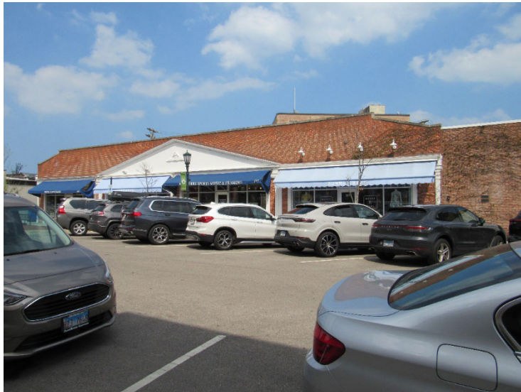
555-571 Chestnut Street (commercial building to west)
