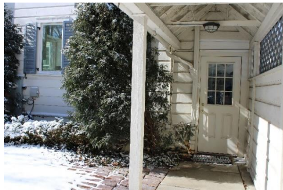
Side door, east façade.
