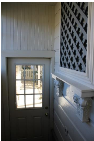
East entrance vestibule.
