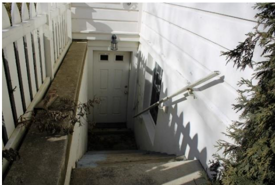
Basement door, east façade.
