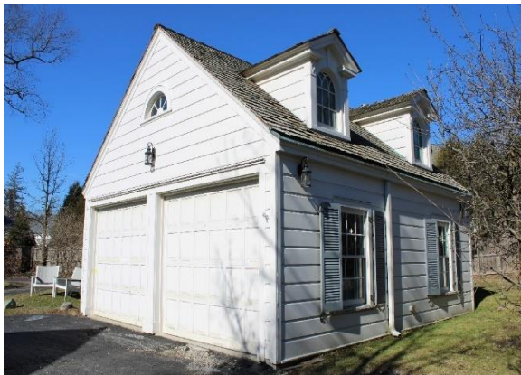
North garage, view northwest.
