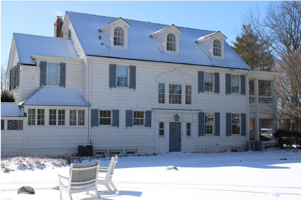
Built 1916-17 Architects Otis and Clark (William Otis and Edwin H. Clark)
