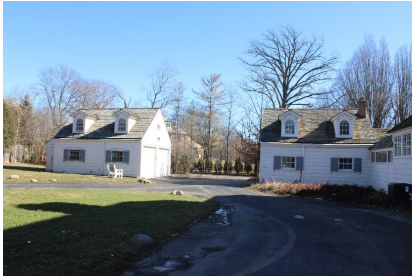
North (left) and south (right) garages, view east.
