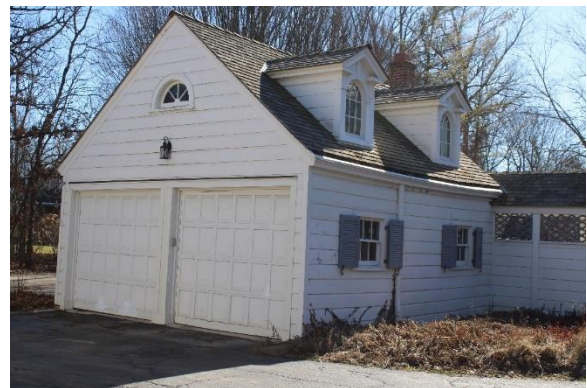
South garage, view southeast.
