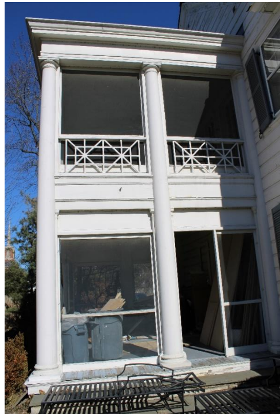
South façade of screened-in porches, view north.
