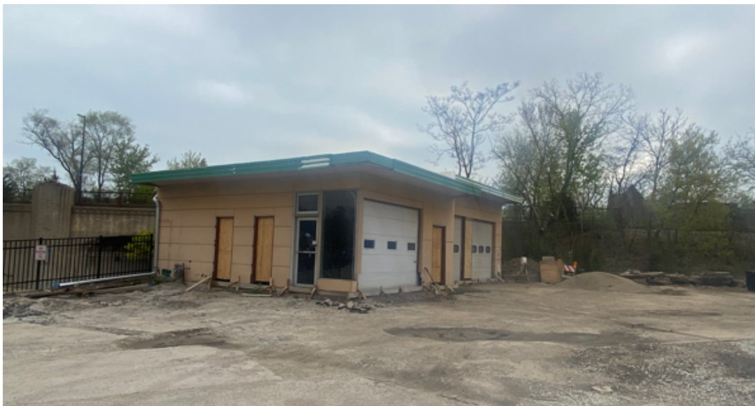
Figure 1 – Subject Property – View from Green Bay Road and Winnetka Avenue intersection
