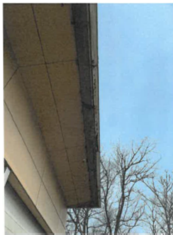
Building fascia with existing lighting along Green Bay Road
