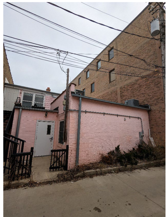
Subject Property – Rear Building Elevation (Alley)
