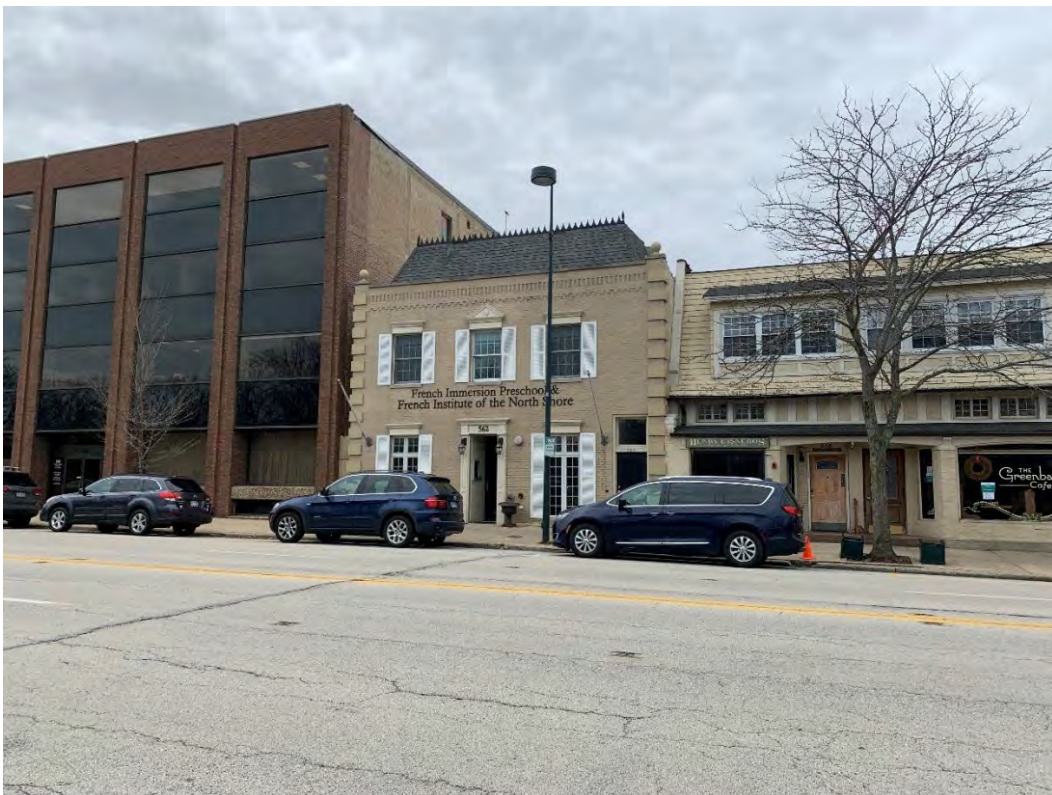
Figure 4 – Subject Property with Neighboring Properties
