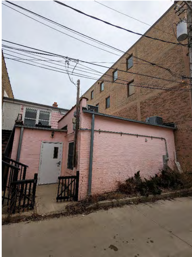
Figure 3 – Subject Property – Existing Rear Building Elevation
