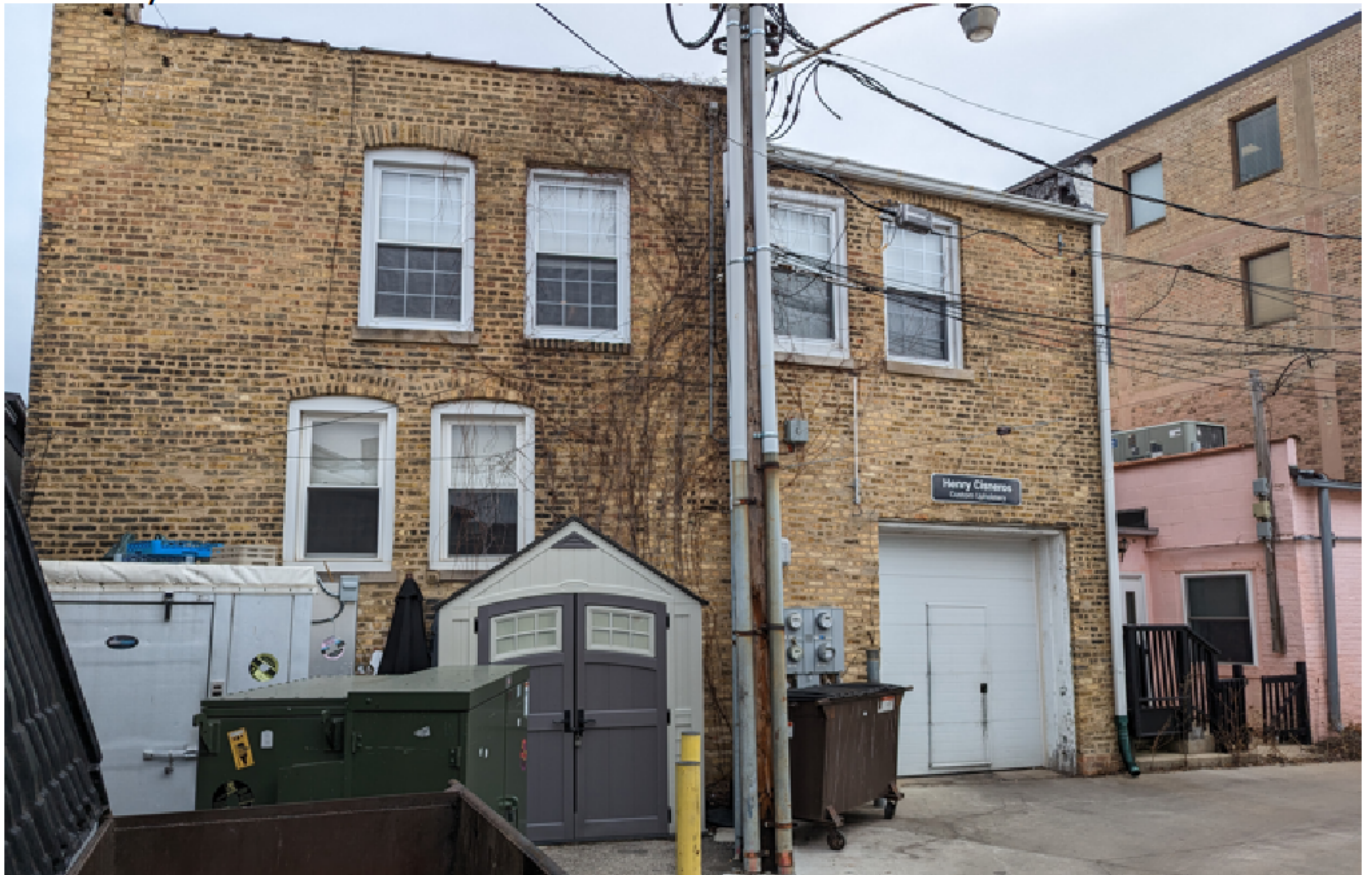
Alley at 560 (North)
