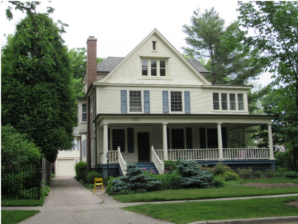
Figure 3 – Subject Property - Front Elevation (Elm Street)
