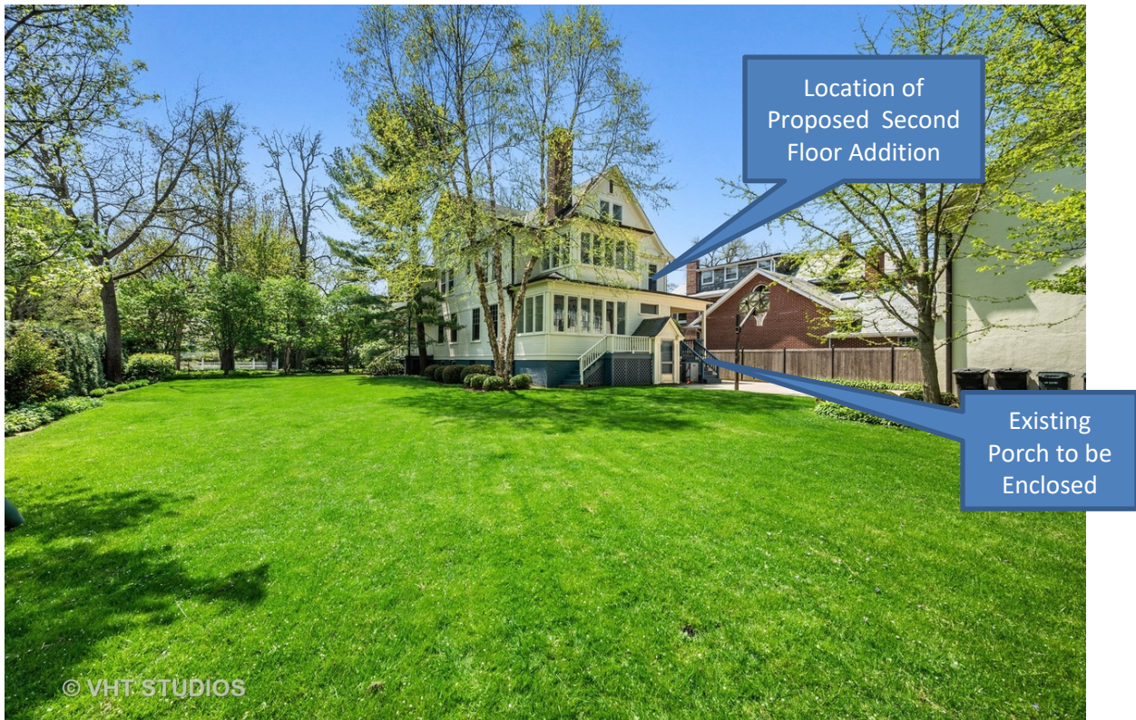
Figure 4 – Subject Property – Rear Elevation
