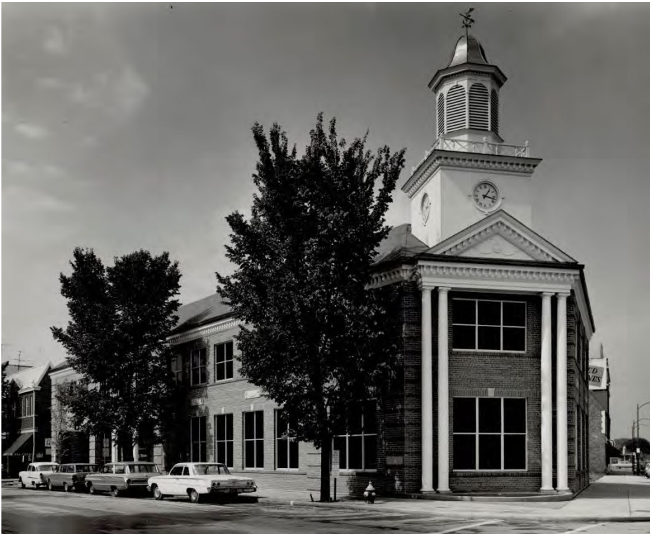
Current bank building at 791 Elm, c. 1964. WHS Collections.
