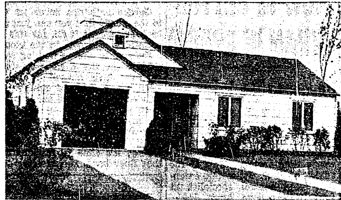
Exterior of the Popular Home house at the Chicago Fair of 1950. It is covered with white asphalt siding. Designed to fit a city lot, it has recreation areas and privacy at the rear.
