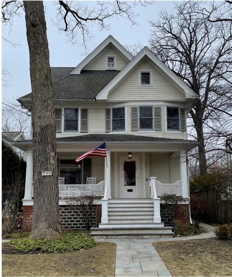
Figure 3 – Subject Property - Front Elevation (Ridge Avenue)
