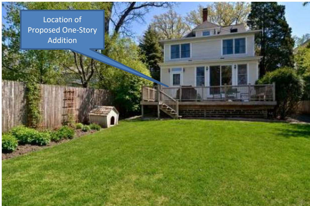
Figure 4 – Subject Property - Rear Elevation
