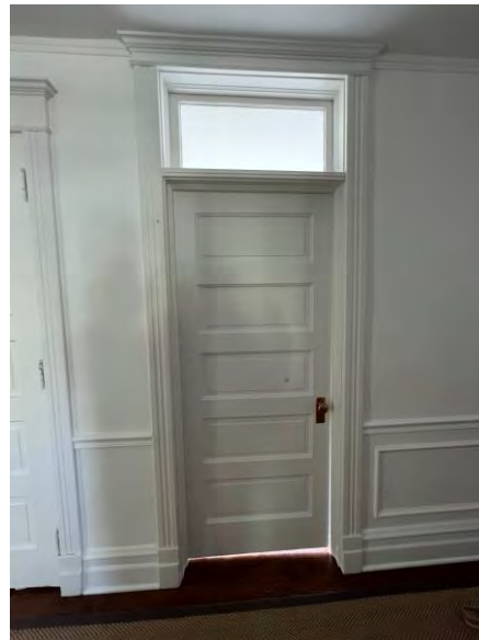
Second floor hall looking west
