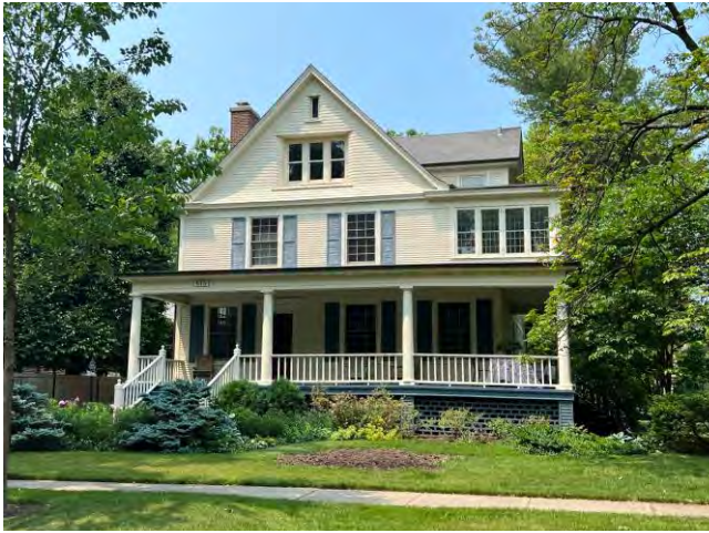
South (front) facade
