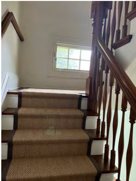
Stairs to 3rd floor
