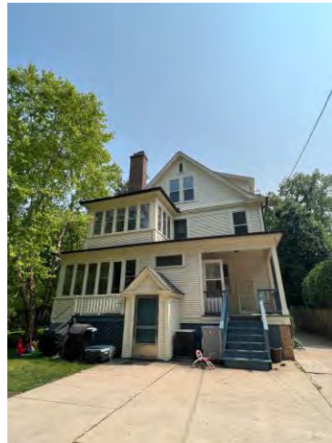
North (rear) facade
