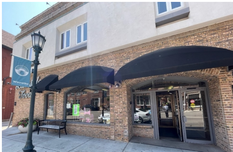
Figure 1 – Subject Property – Store frontage of Lakeside Foods along Elm Street
