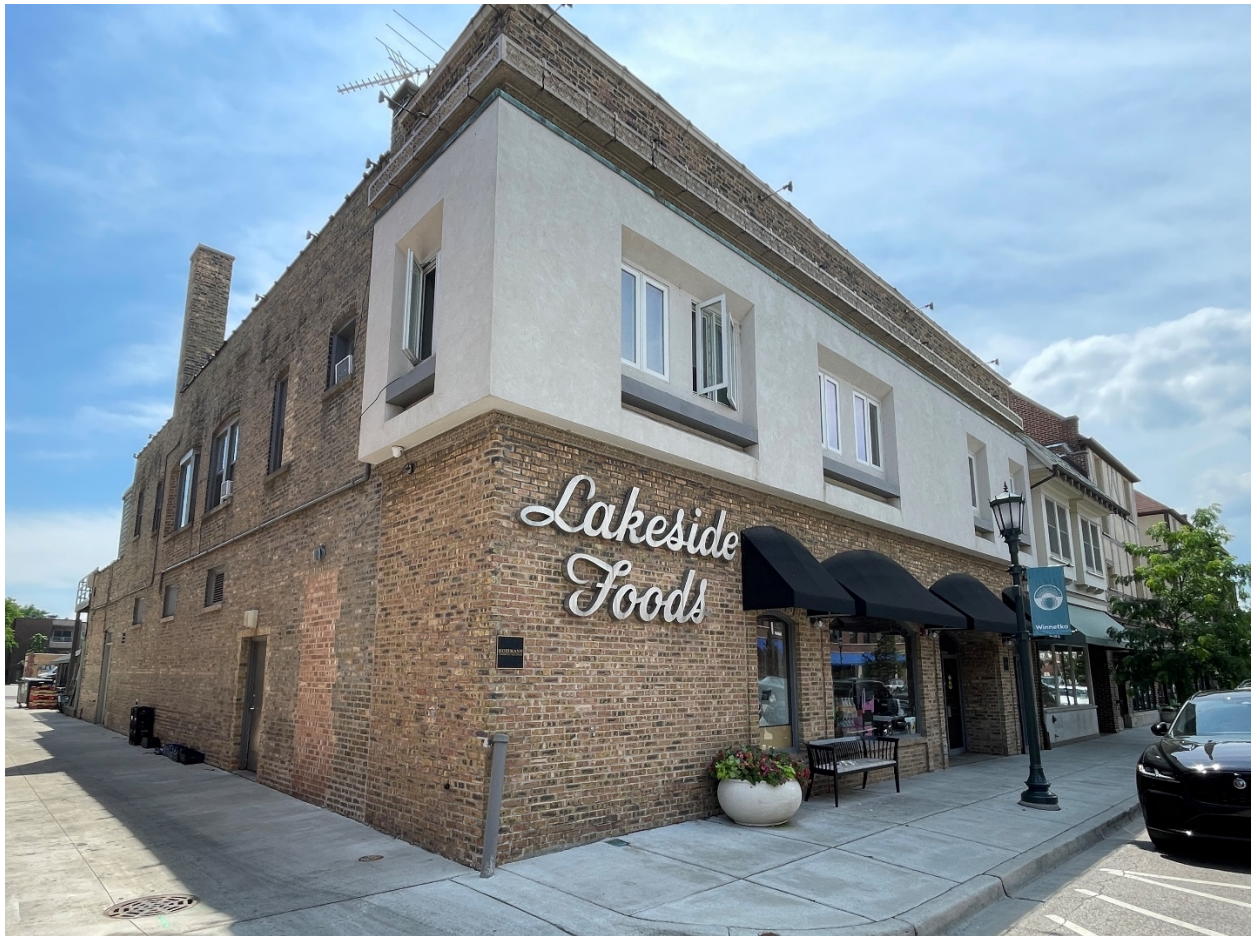
Figure 4 – Subject Property – Corner of main storefront along Elm Street, facing southwest
