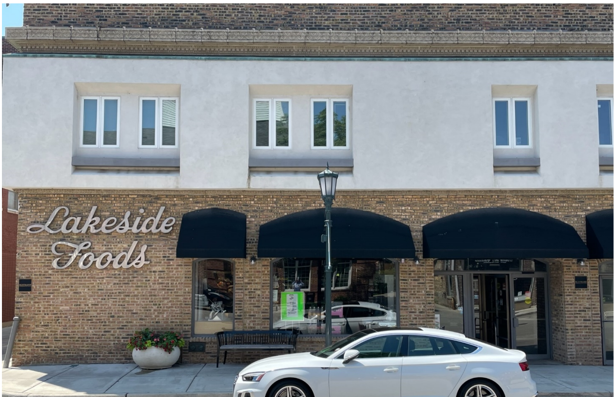
Figure 5 – Subject Property – Storefront façade along Elm Street
