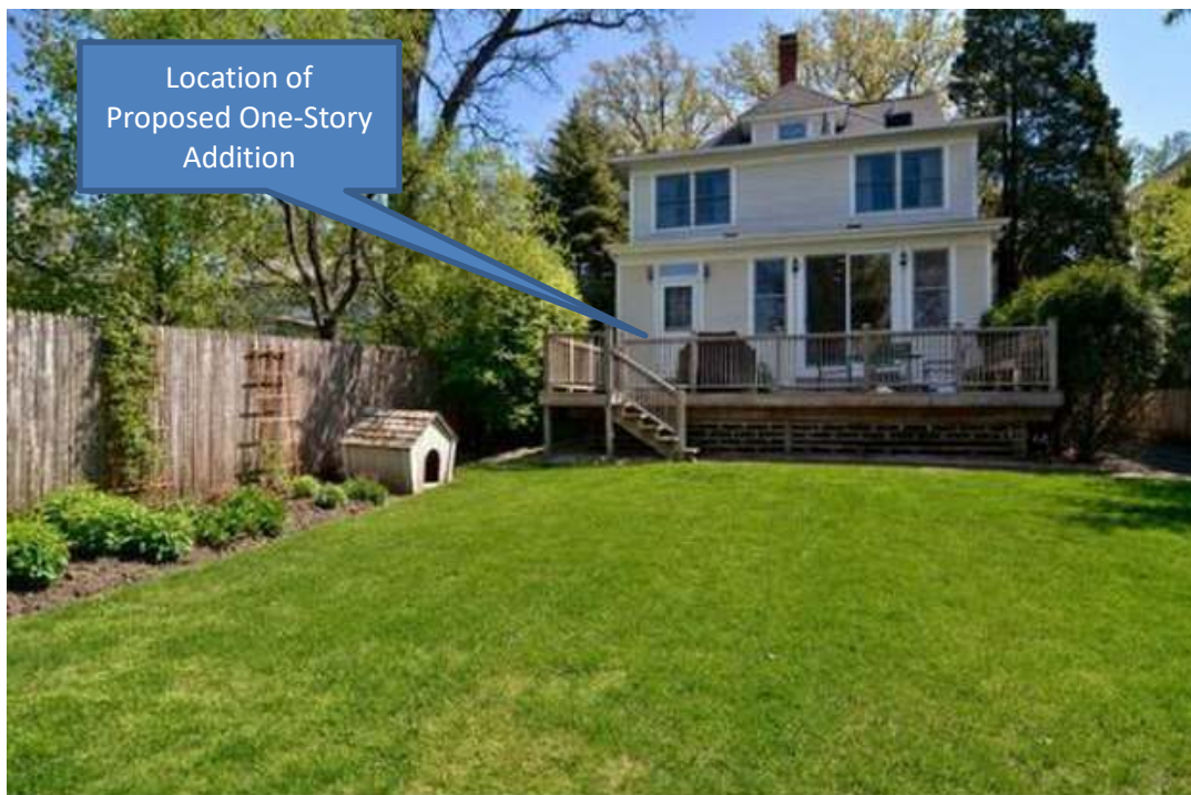
Figure 4 – Subject Property - Rear Elevation
