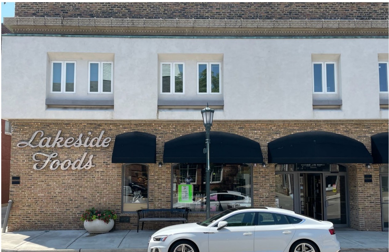
Figure 5 – Subject Property – Storefront façade along Elm Street
