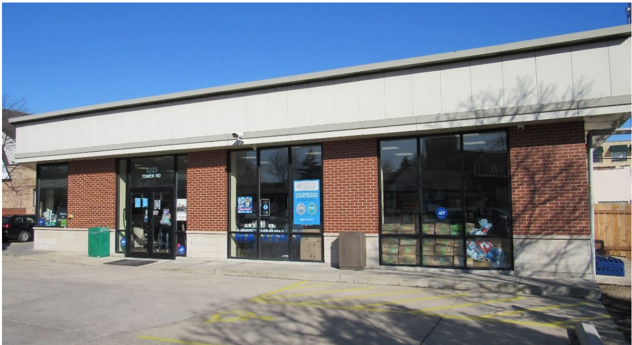
Figure 3 – Subject Property – South building façade along Tower Road
