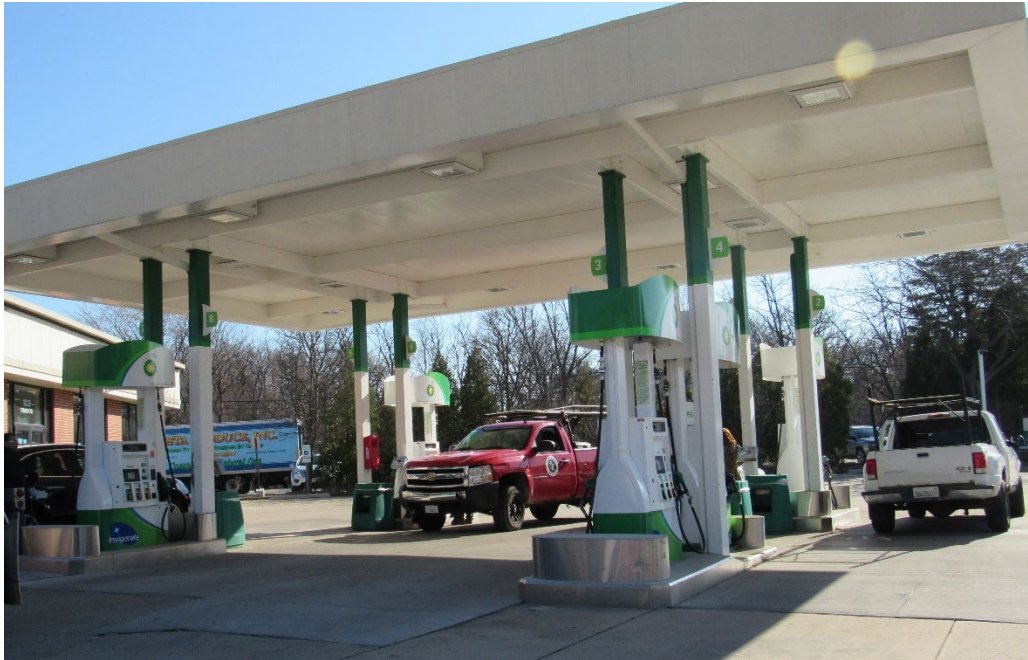
Figure 4 – Subject Property – Gas pump canopy structure along Tower Road
