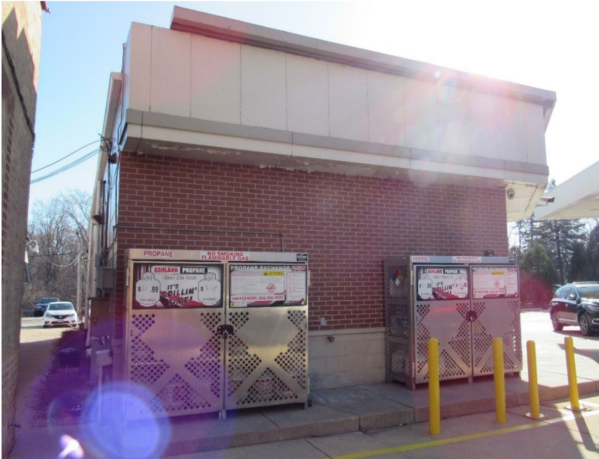
Figure 2 – Subject Property – West building façade along Green Bay Road
