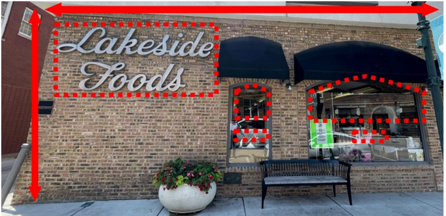
Lakeside Foods – Elm Street Frontage
