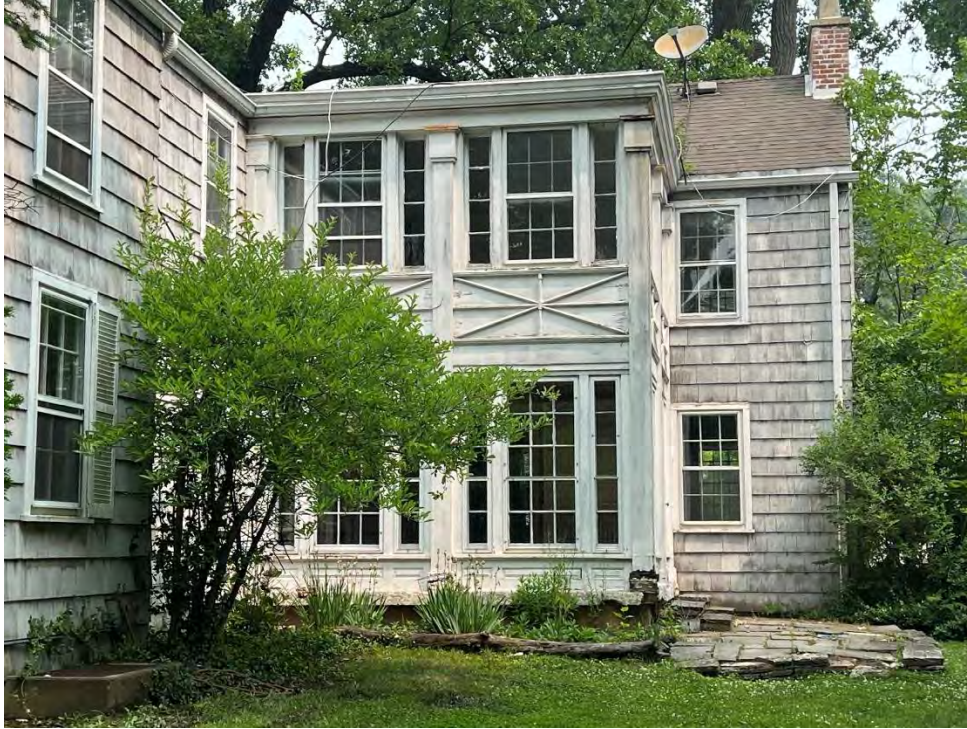
South facades, East End. Sunrooms
