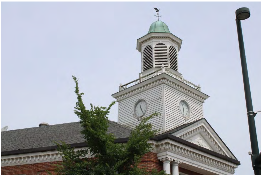
Detail of cupola, view north.
