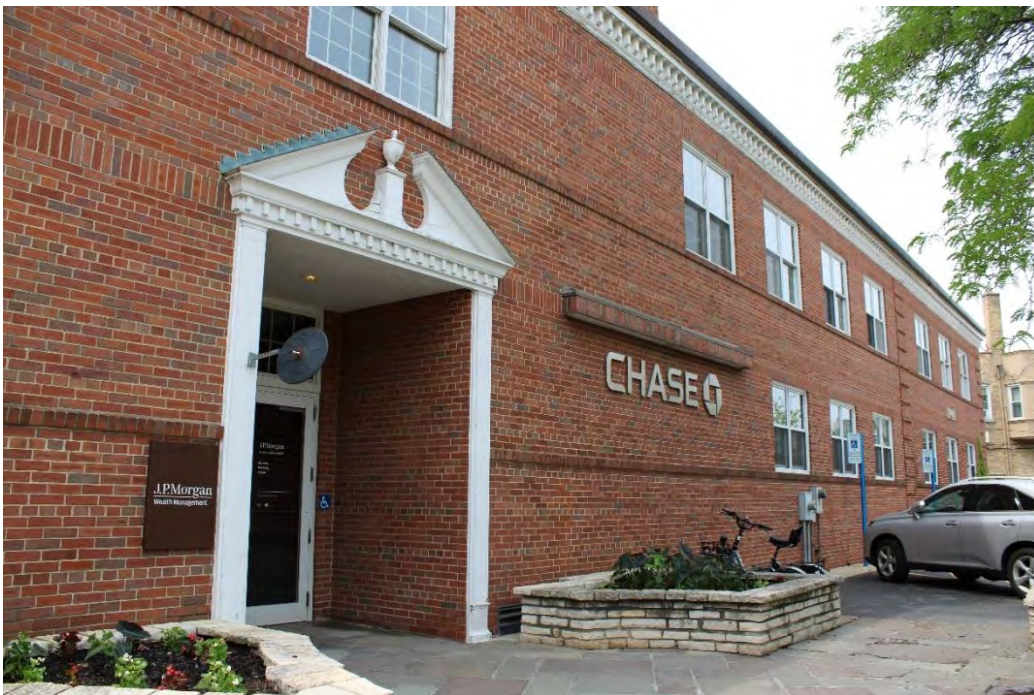
North façade, view southwest.
