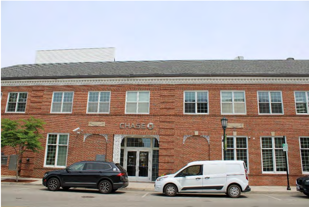
South façade, view north.
