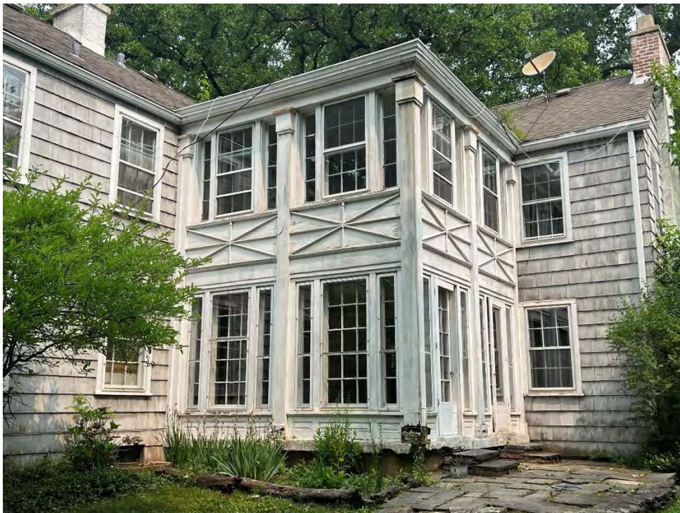
Inside, Southeast corner, Sunrooms
