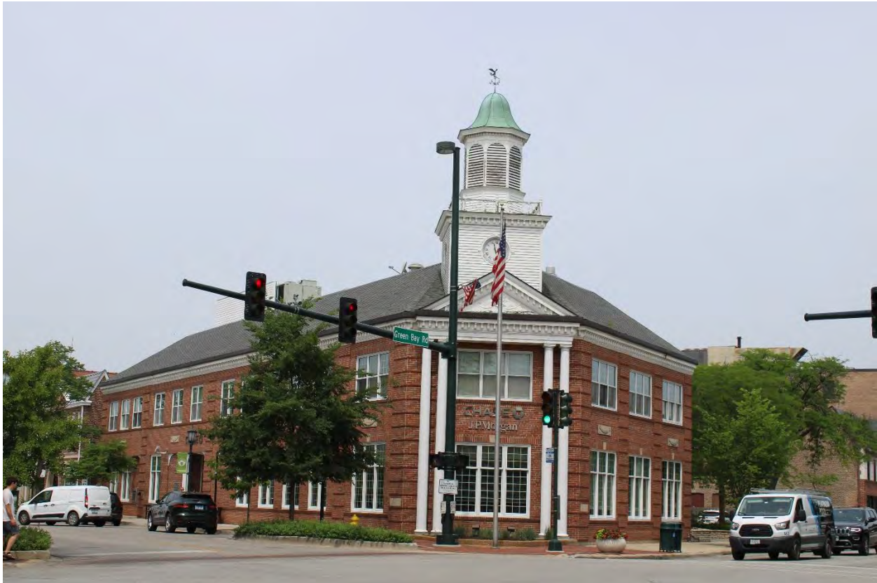
Built 1963-64 Architect Peter Mayo of the firm Mayo and Mayo
