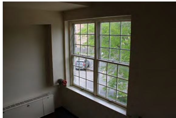
Interior view of windows.
