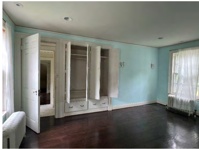
Second Floor West-Center Bedroom
