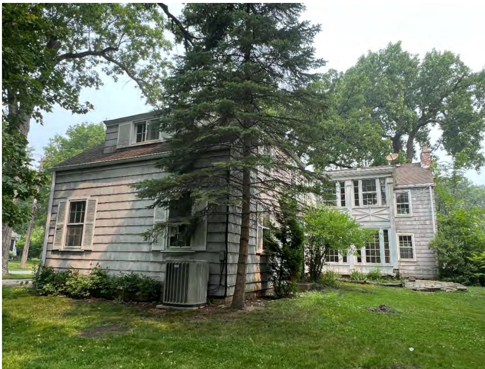
East Facades: Garage. Sun Rooms
