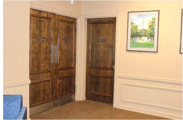
Basement wood doors.
