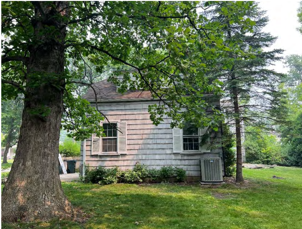
South Façade, Garage
