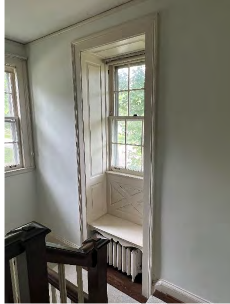
Main Staircase, Landing
