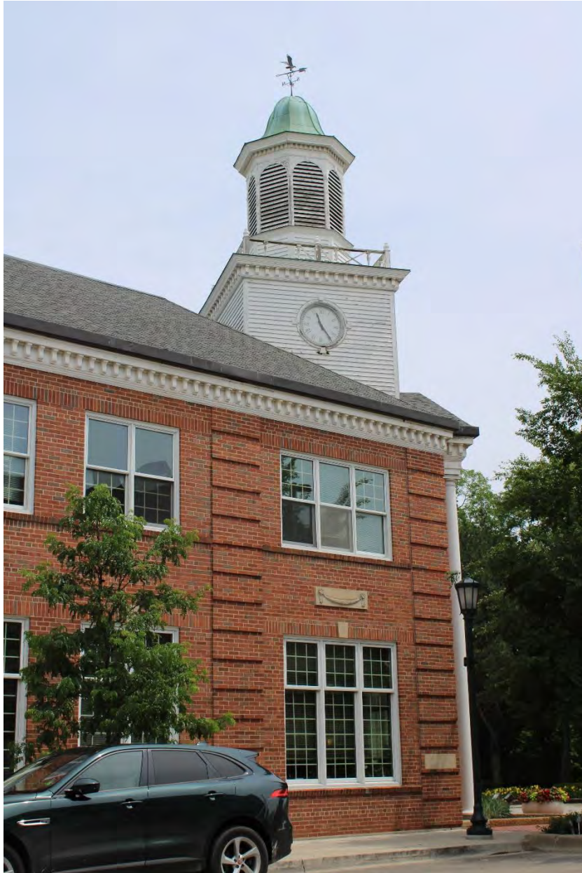
Detail of south façade, view north.
