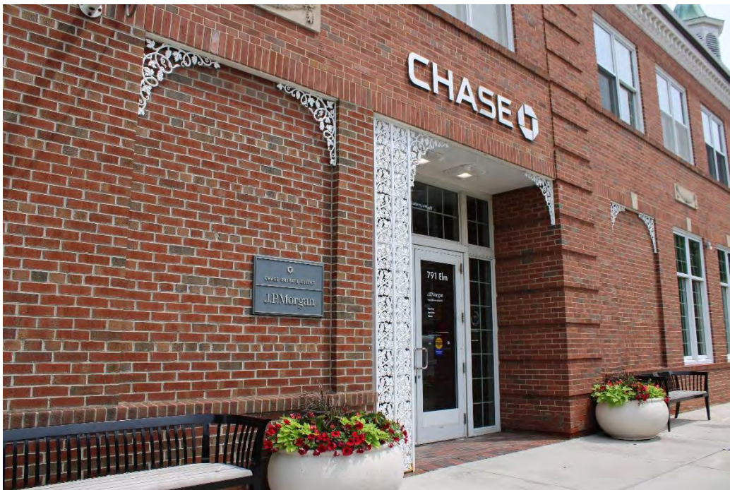
Detail of south façade entrance.
