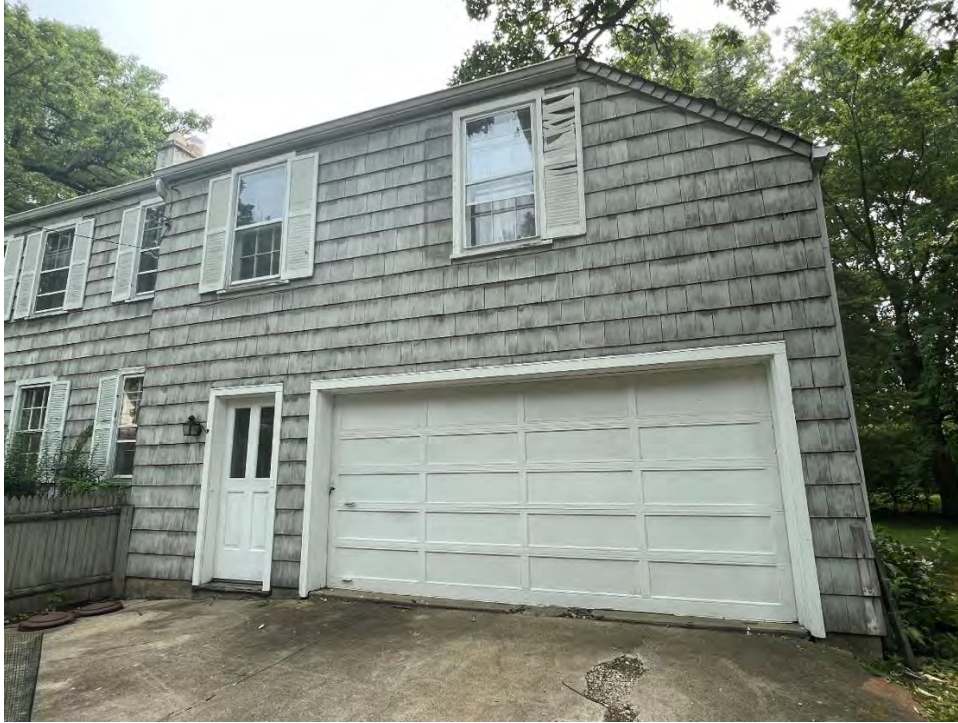
West Façade, South End, Garage
