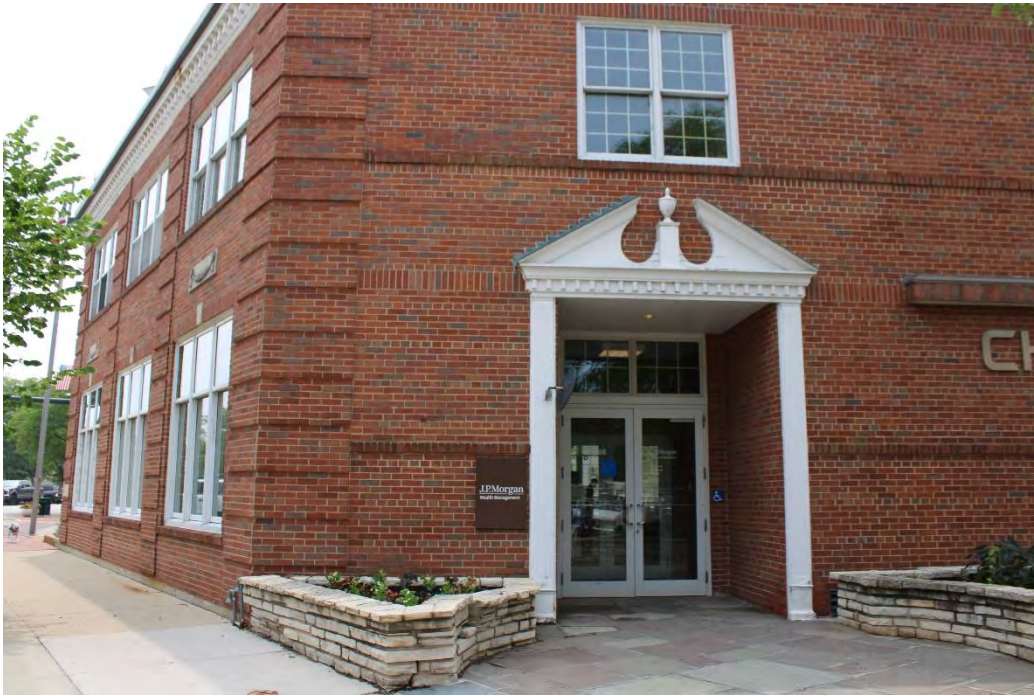
North entrance, view south.
