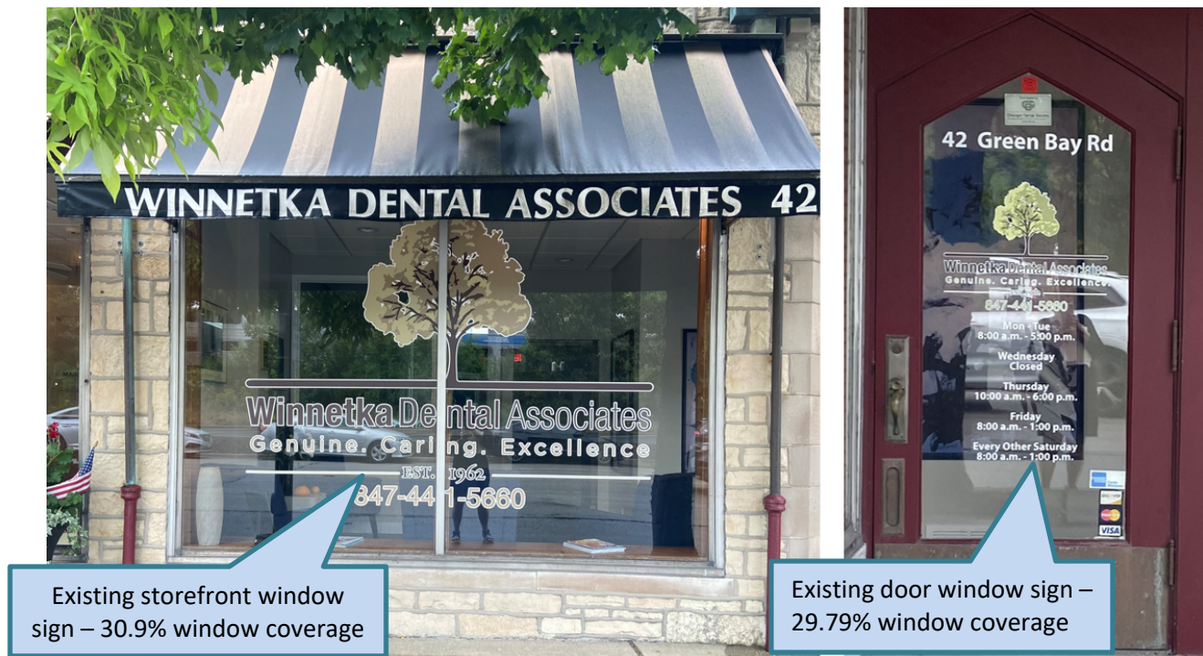
Figure 3 – 42 Green Bay Road - Storefront with existing window and door signs
