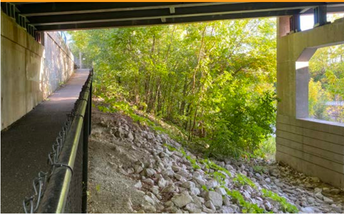
View of ramp access under Pine St. bridge
