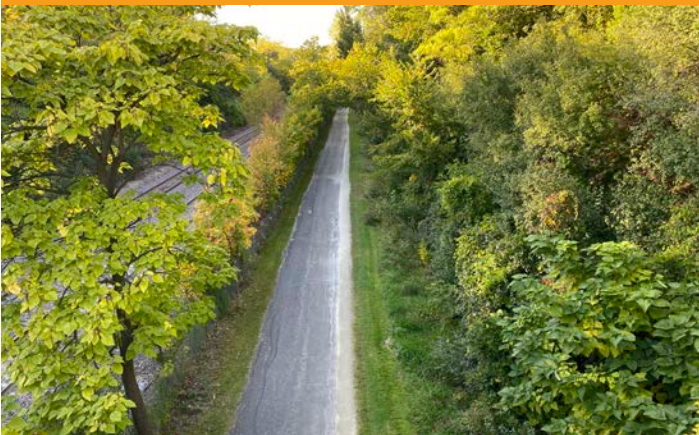
View of trail looking north at Eldorado St. bridge
