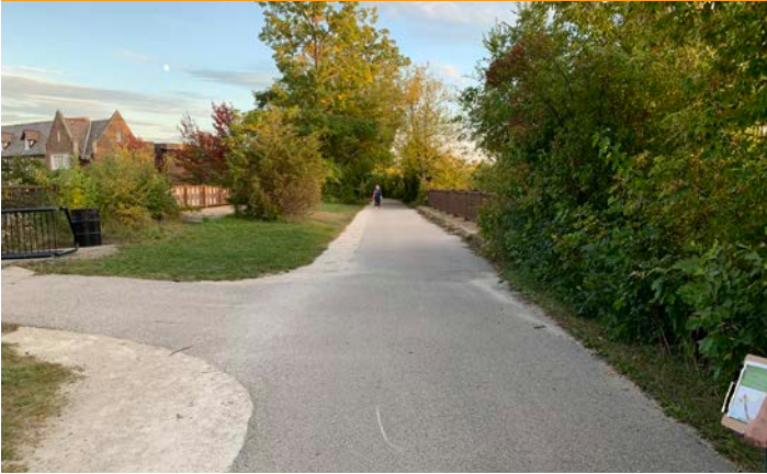
View of trail looking south at Winnetka Ave. bridge
