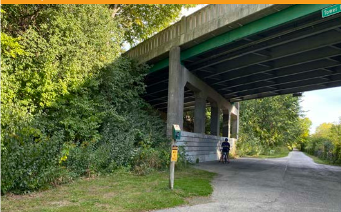
View of trail looking south at Tower Rd. bridge
