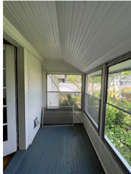
Second floor porch looking north
