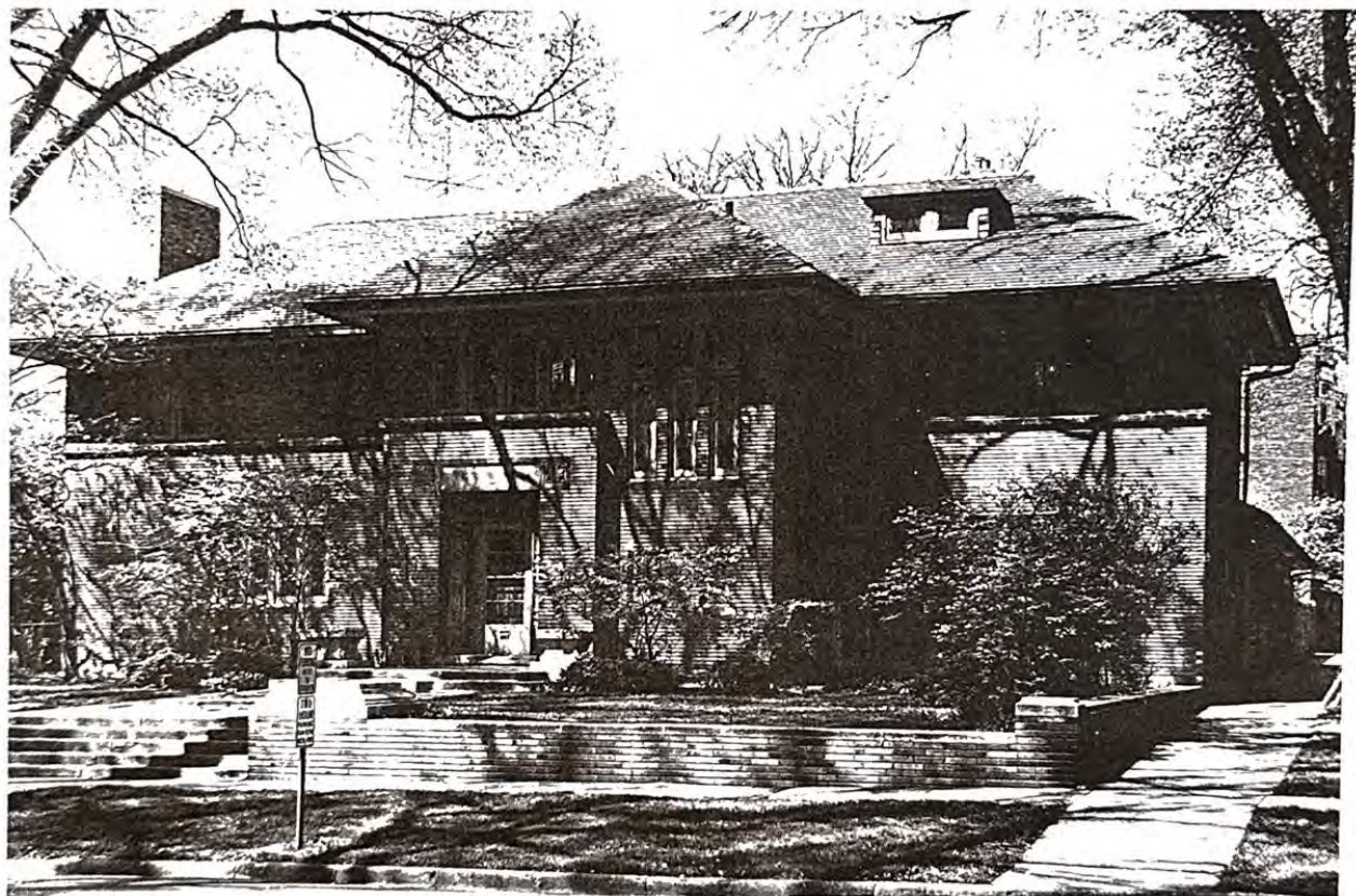
FIG. 38 Spencer and Powers. Edward W. McCready house, 231 N. Euclid Avenue, Oak Park, Illinois, 1907. Historic American Building Survey photo by Richard Nickel
