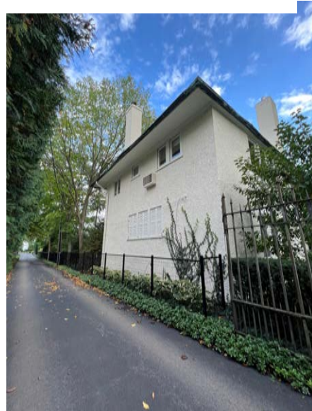
North façade looking east
