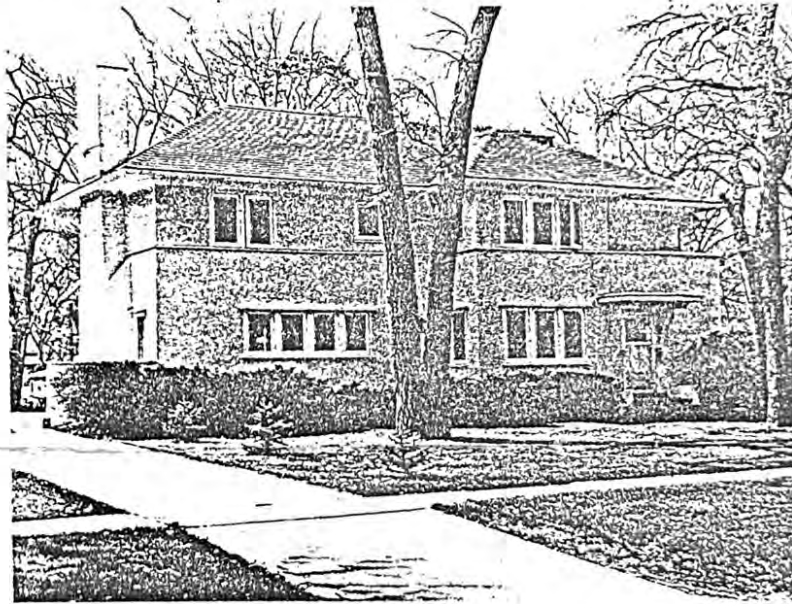
FIG. 37 Robert C. Spencer, Jr. Robert C. Spencer, Jr house, 926 Park Avenue, River Forest, Illinois, 1905. Photo by H.A. Brooks
