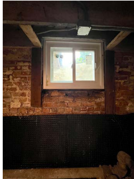
Basement looking south
