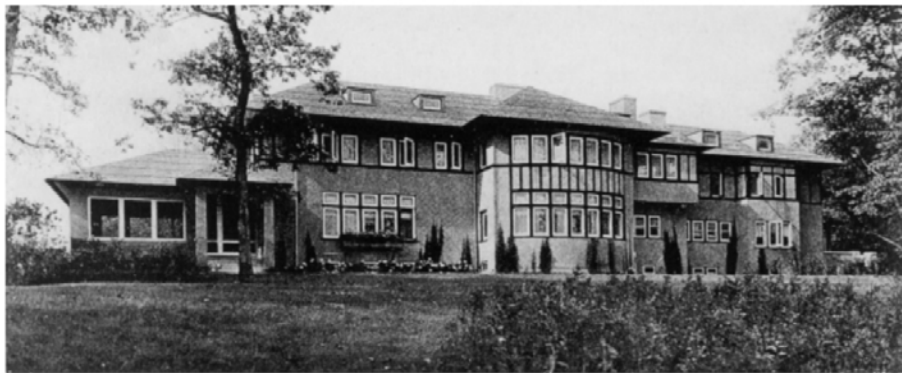
Fig. 2. Robert C. Spencer, Jr., A. C. Magnus house, Winnetka, Ill., 1904. From Western Architect 20, no. 4 (April 1914). East facade, facing Lake Michigan.
