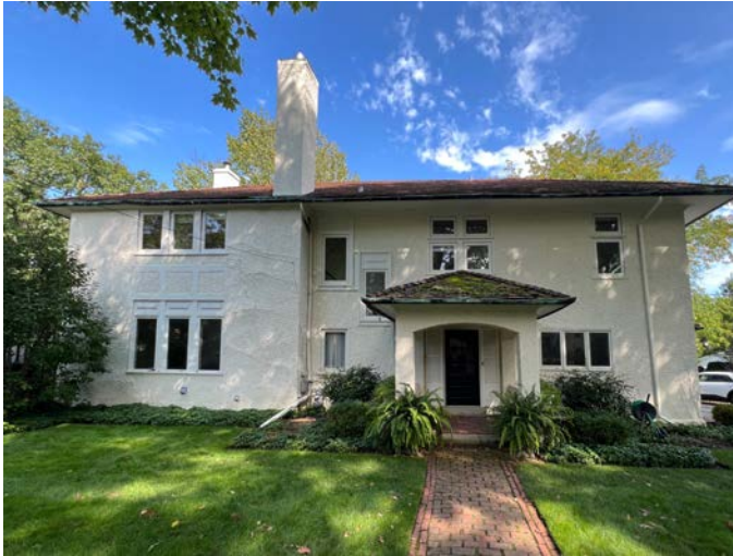
Front (west) facade
