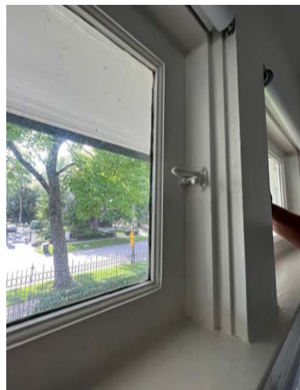
South bedroom window hardware
