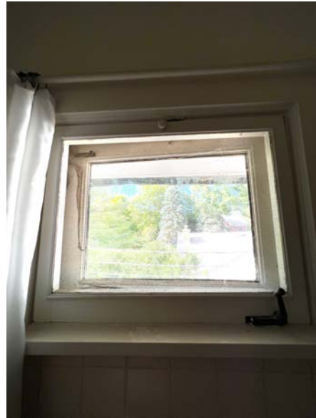
Second floor window
