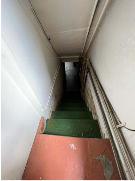
Stairs to basement from inside mechanicals room
