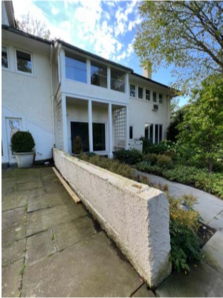
East façade looking northeast
