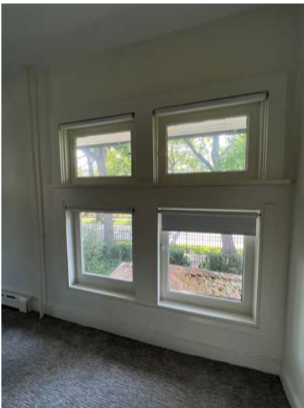
South bedroom windows
