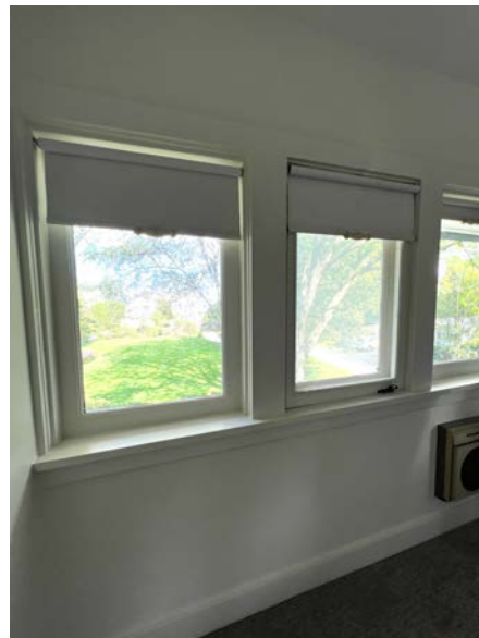
South bedroom east wall windows
