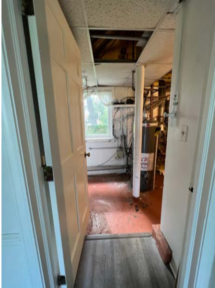
Mechanicals room looking west
