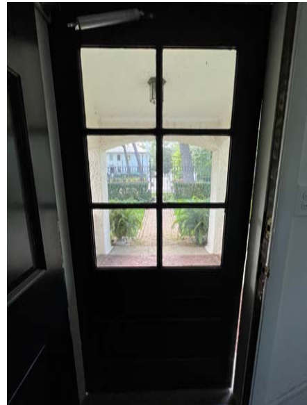
View through front entry looking west
