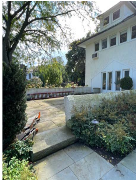
East façade looking south, site of former greenhouse
