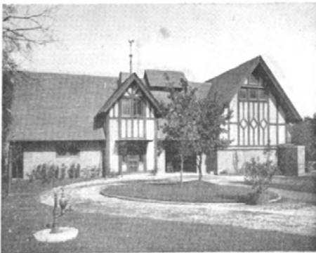
Mr. U. S. Orendorff's Barn, Canton, Ill. R. C. Spencer, Jr., Architect
