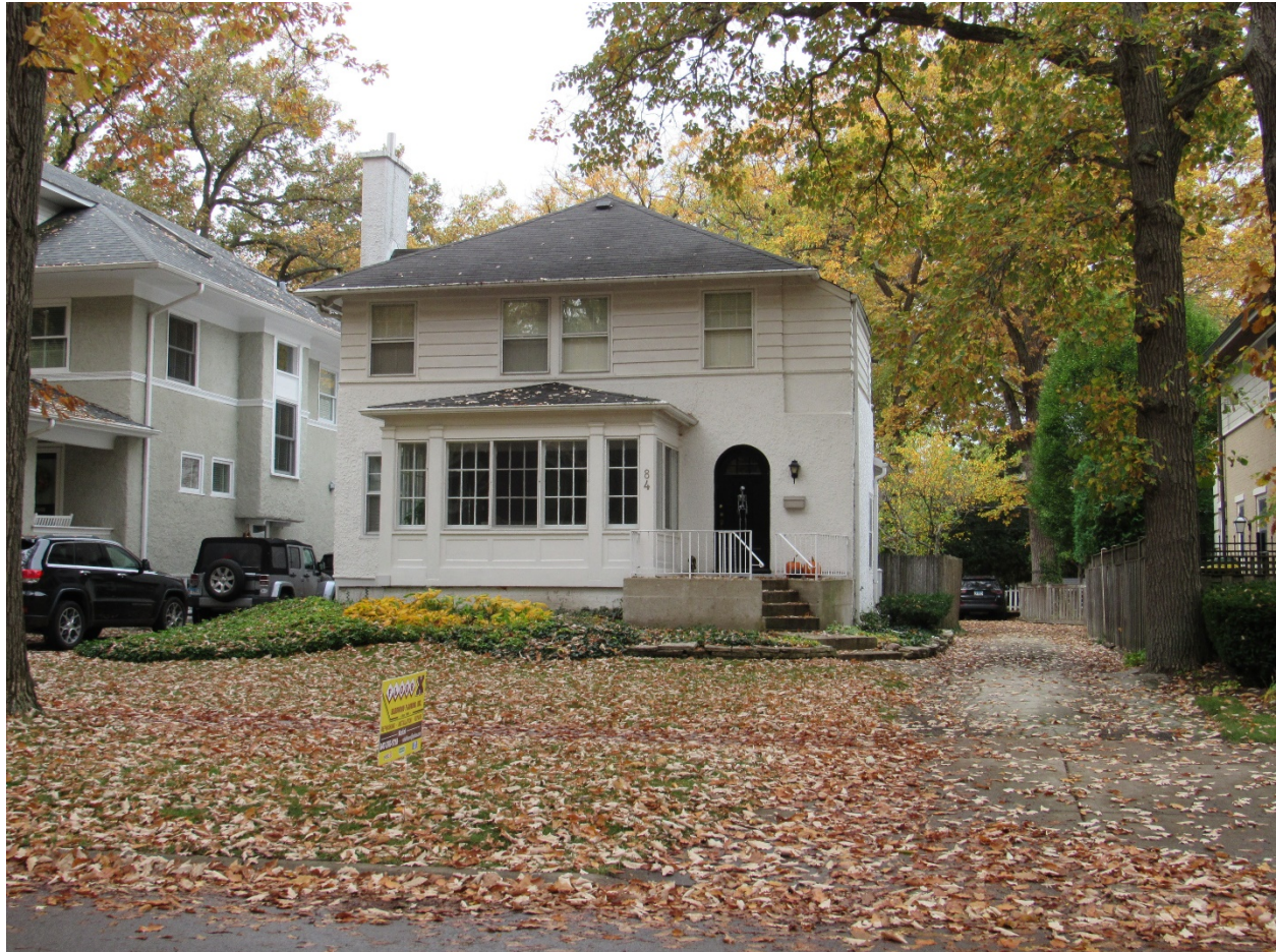
Figure 4 – Subject Property (Front Elevation – Abbottsford Road)
