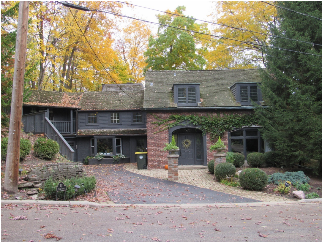
Figure 5 – Subject Property (Front/South Elevation – Park Avenue)
