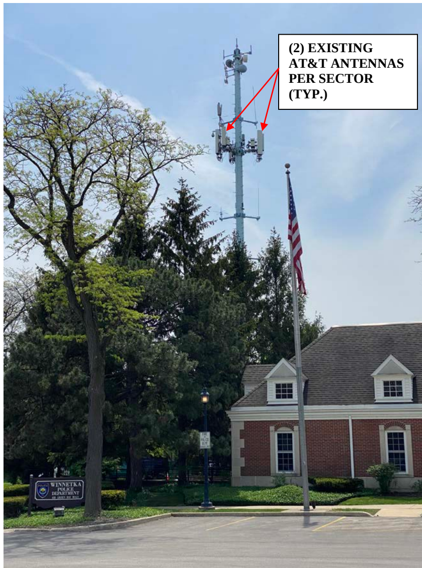
NORTH ELEVATION BEFORE
