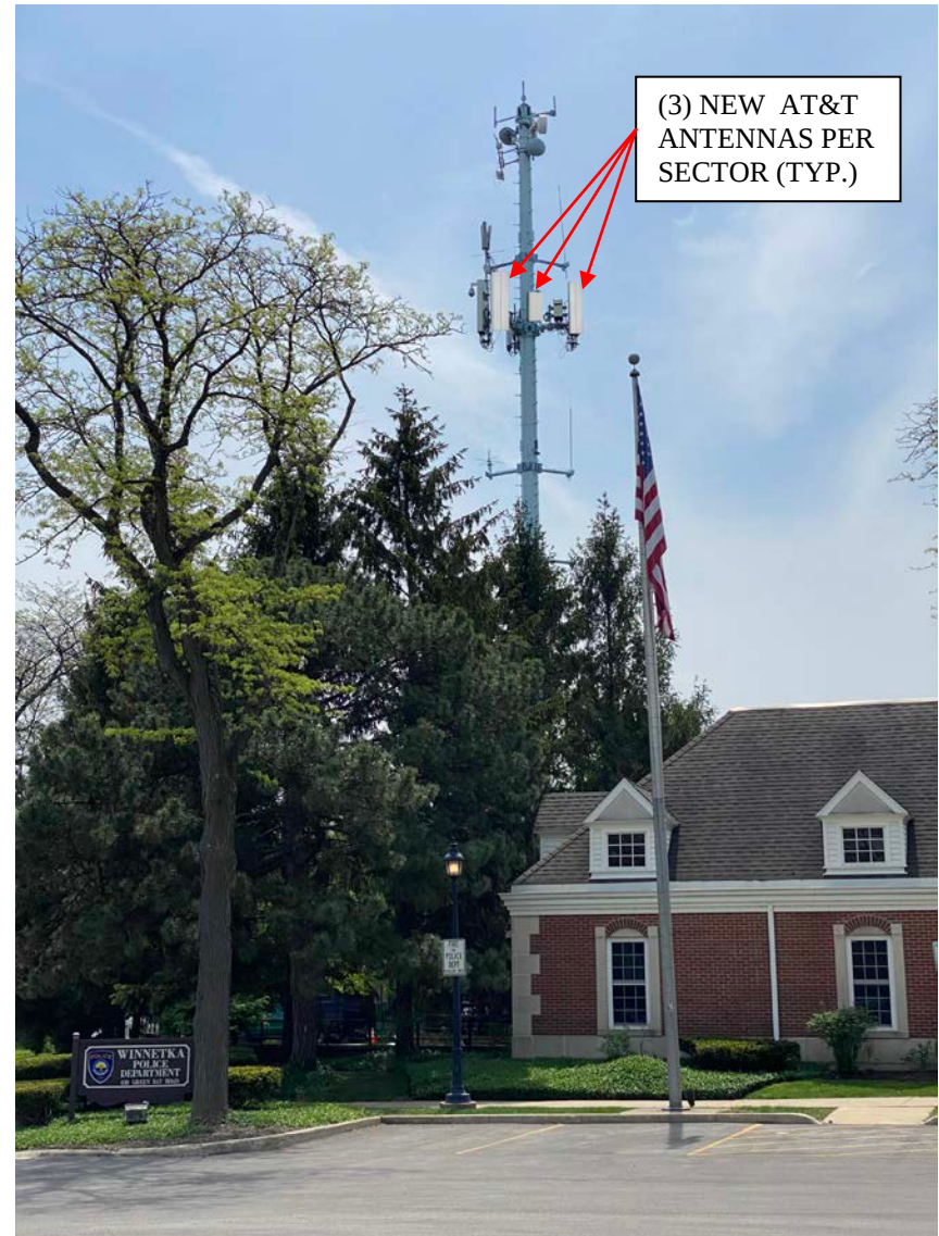
NORTH ELEVATION AFTER
