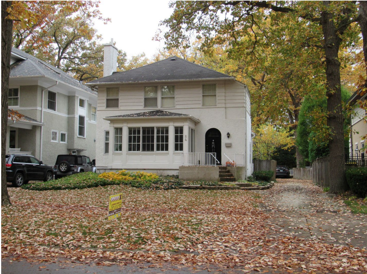
Figure 4 – Subject Property (Front Elevation – Abbottsford Road)
