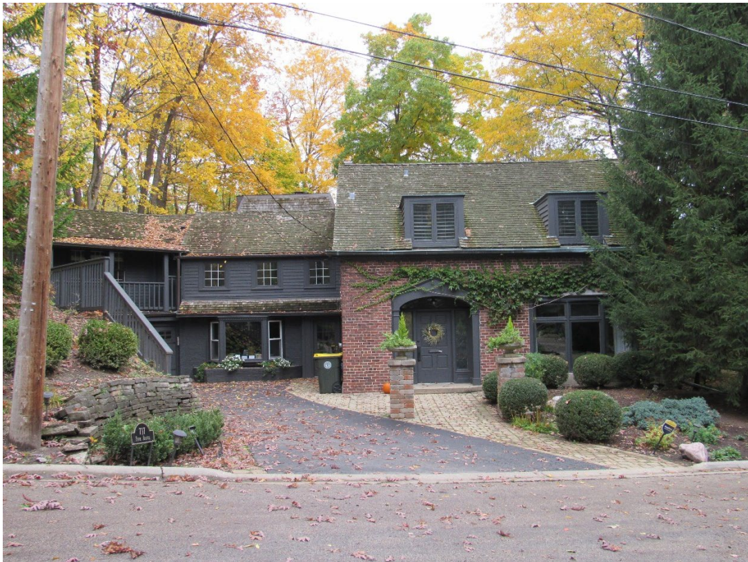
Figure 5 – Subject Property (Front/South Elevation – Park Avenue)
