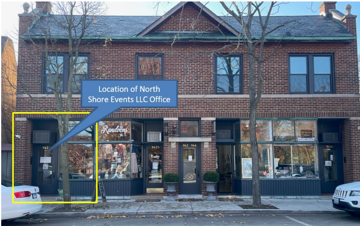
Figure 2 – Subject Property – 962 Green Bay Road
