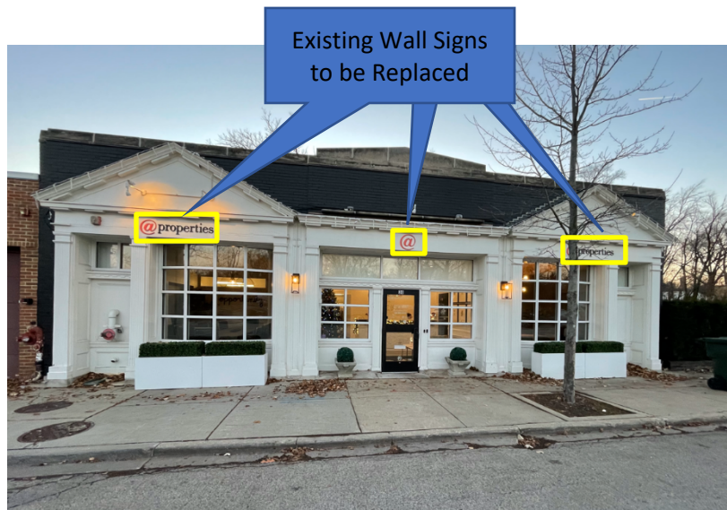
Figure 2 – Subject Property – Building View/along Green Bay Road
