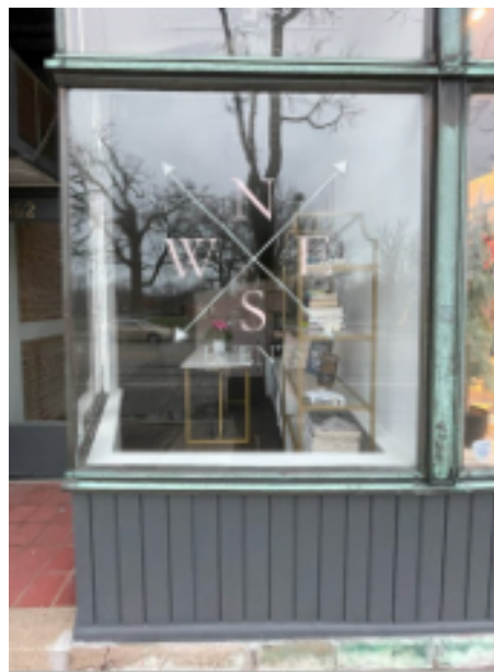
962 Green Bay Road – Recently installed storefront window sign
