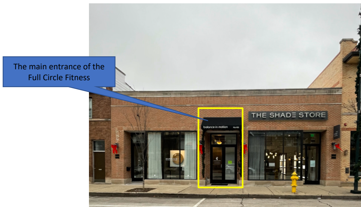
Figure 1 – Subject Property View of the entire building from Green Bay Road
