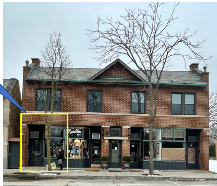
Figure 1 – Subject Property View of the entire building from the Green Bay Road
