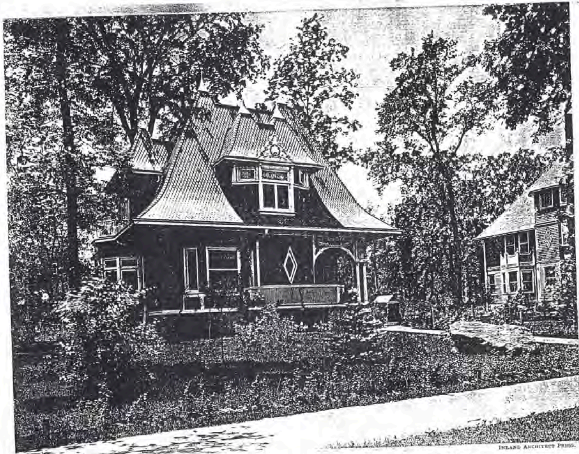
RESIDENCE OF GEO. W. MAHER, KENILWORTH, CHICAGO. GEO. W. MAHER, ARCHTCT.
