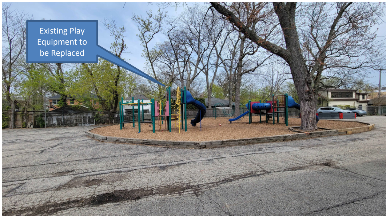
Figure 5 – Subject Property - Playground – Looking North
