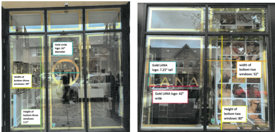
Subject Property – Storefront door and window signs recently installed
