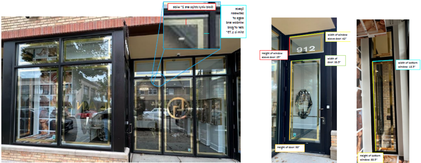
Subject Property – Storefront with recently installed vinyl gold border/ribbons around doors & windows
