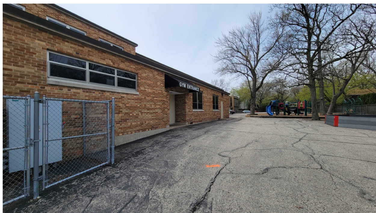
Figure 6 – Subject Property – Looking West
