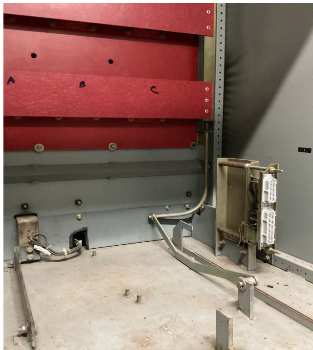
5.11 FPE Breaker cubicle – Stationary secondary contacts
