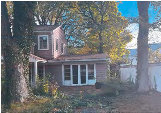
South façade looking east
