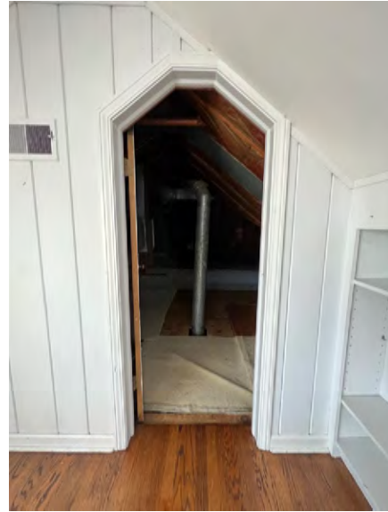
Second floor attic space
