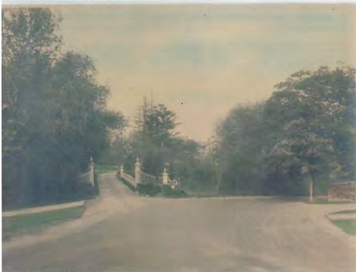
Entrance Gate to Estate, 1933
