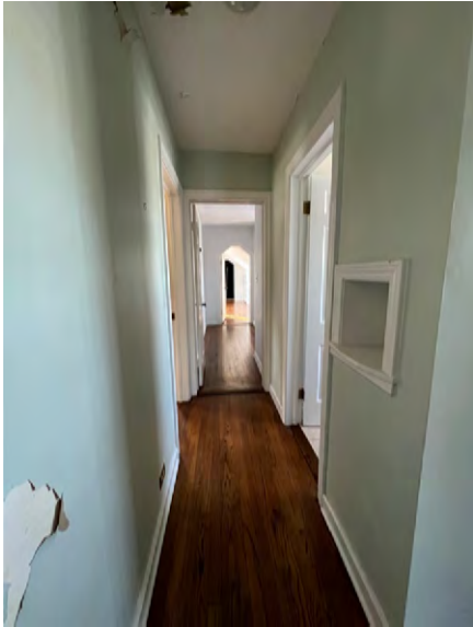
Second floor hall looking west
