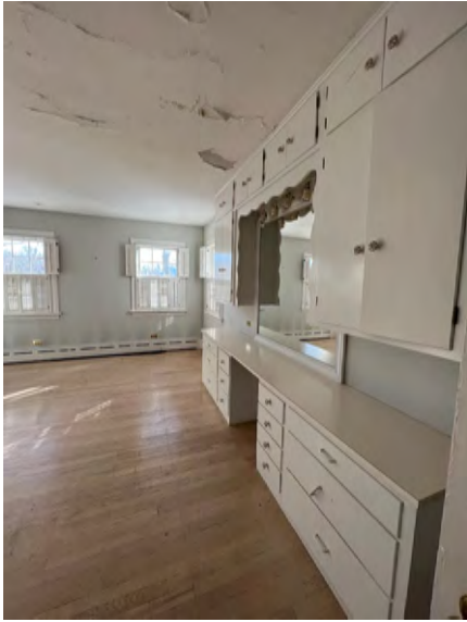
Second floor southeast bedroom
