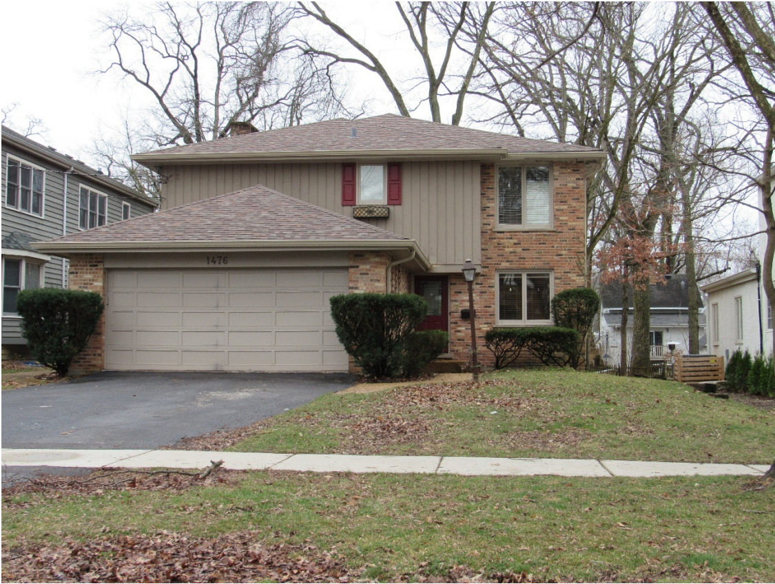
Figure 3 – Subject Property - Front Elevation (Scott Avenue)
