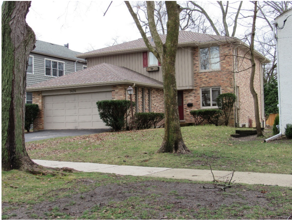
Figure 5 – Subject Property (West Elevation)
