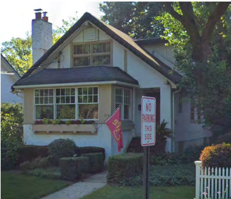
Lloyd and Margaret Faxon House, 228 Poplar Street, 1919
