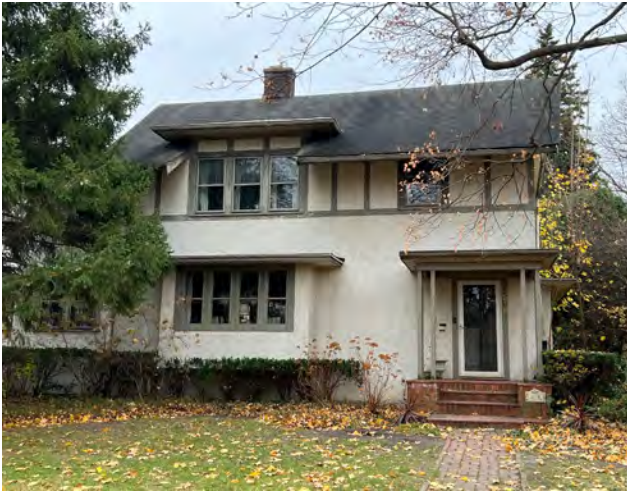
Front (north) facade
