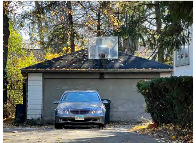
Garage, north facade
