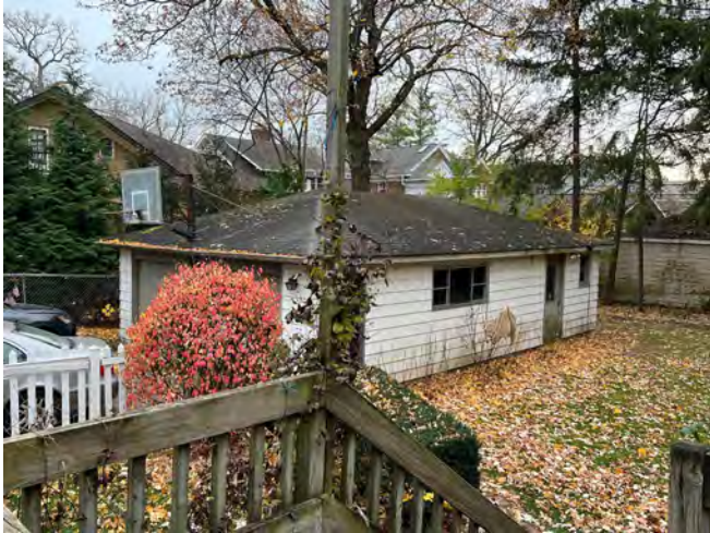
Garage, view from rear deck
