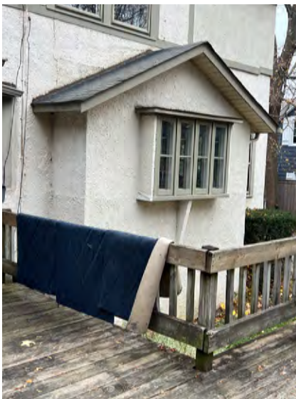
Rear bay and deck
