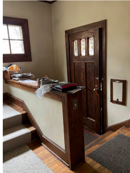
Front hall view toward front door
