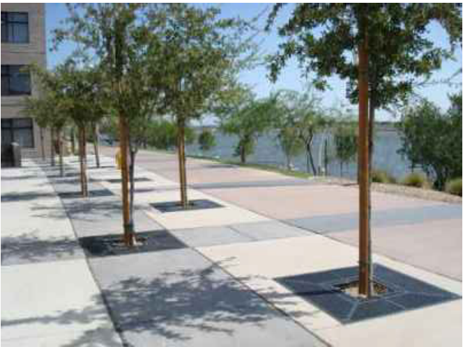
PLAZA TREE IN GRATE NEENAH FOUNDRY MODEL 8704 - 3'x3'
