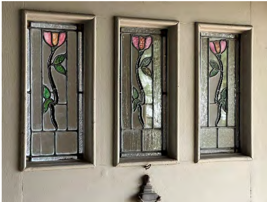
518 Elder Lane, Windows in front door of house, 2023
