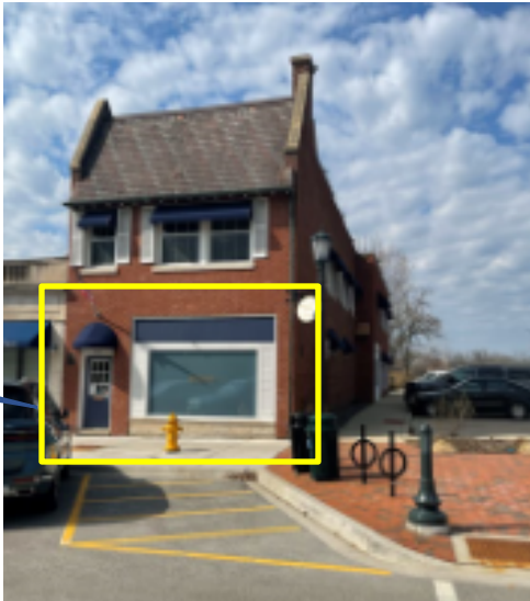
Figure 2 – Subject Property Storefront of the new post office location - View from Lincoln Avenue
