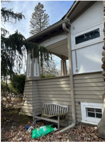
East façade, front porch, looking southwest
