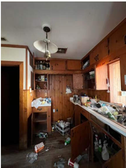
Kitchen looking west, entrance to basement on left
