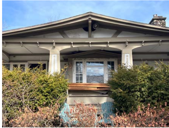
Front (south) façade, looking north
