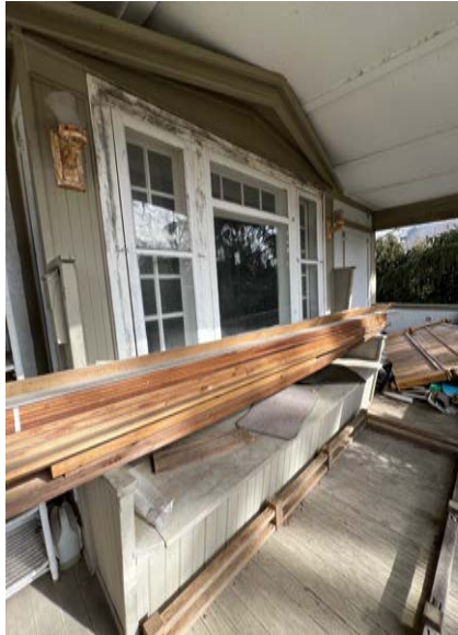
Front porch looking east
