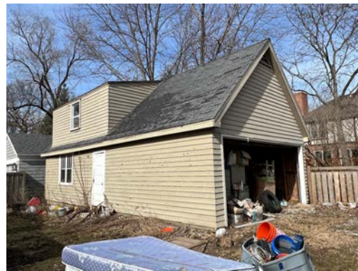
Garage looking northwest
