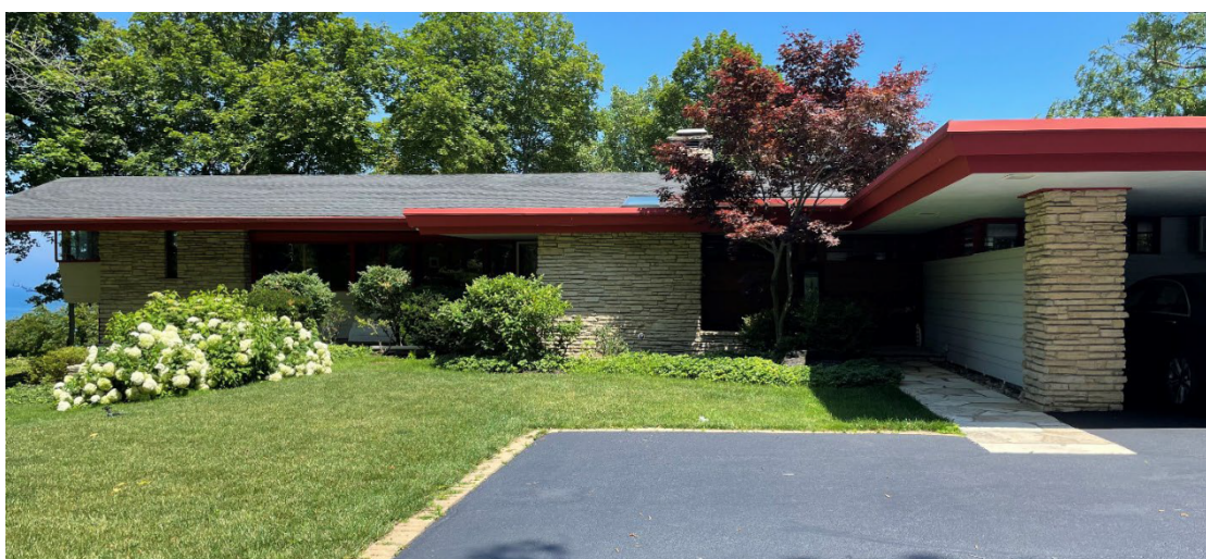
Figure 3 – Subject Property (East Elevation From Driveway)
