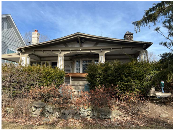
Front (south) façade, looking north
