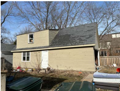
Garage looking north
