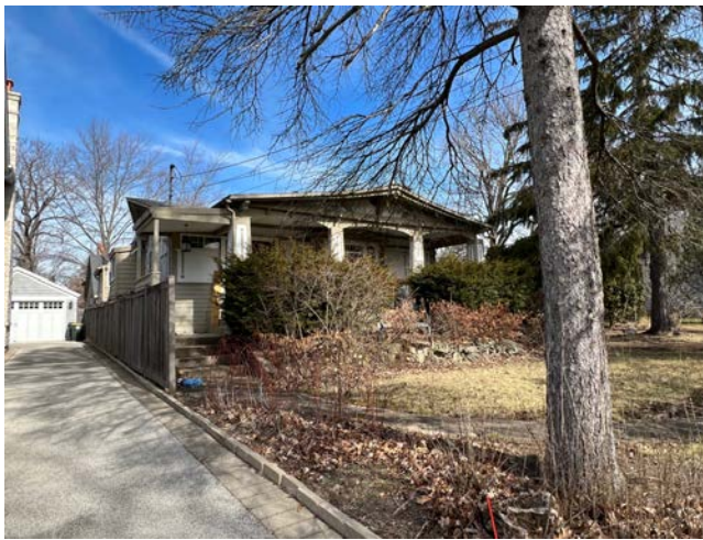
Front (south), east facades
