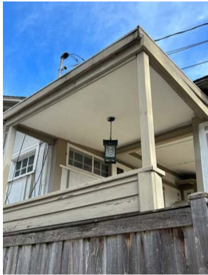
Front porch looking northeast
