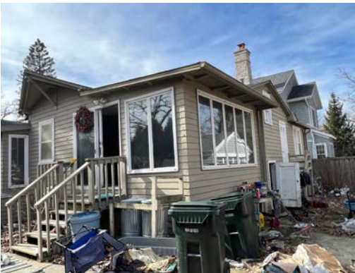
East, north facades looking southwest
