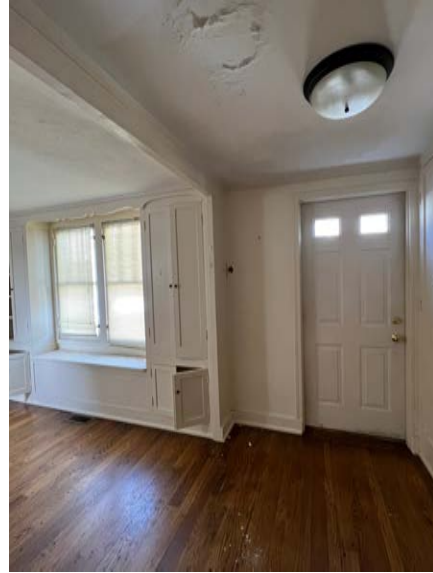
Bedroom 3 looking north
