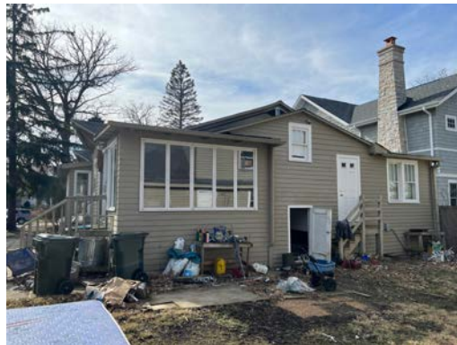
North façade looking south
