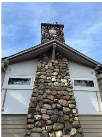
East façade chimney
