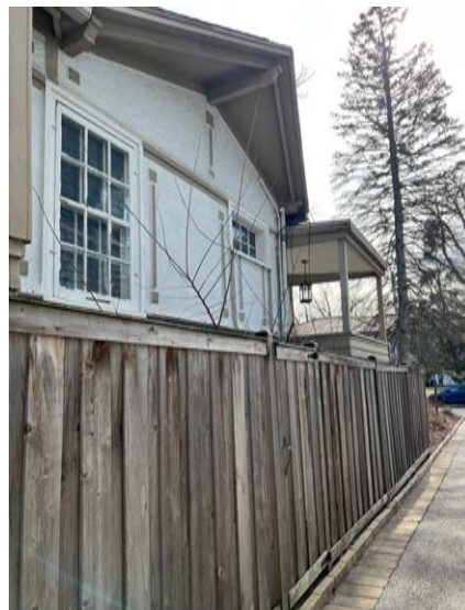
West façade looking south
