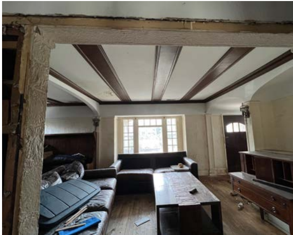
Living room looking south
