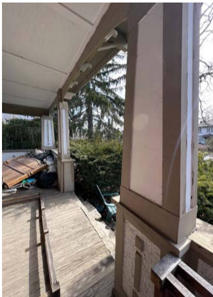
Front porch looking east
