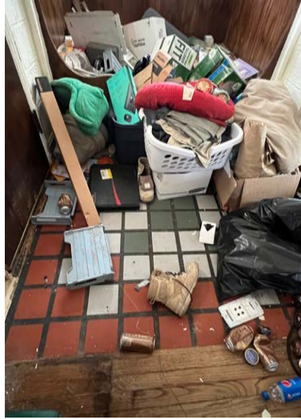
Front entry vestibule tile floor
