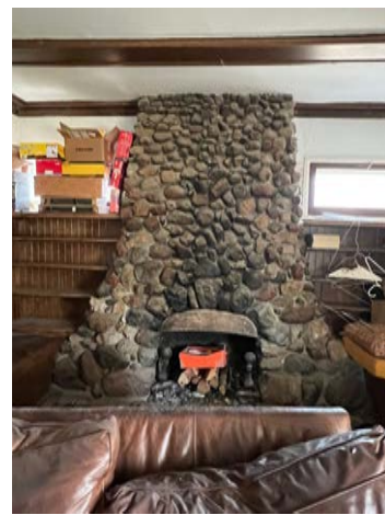
Fireplace, living room looking east
