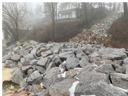
Lloyd Park/Boat Launch outfall.
