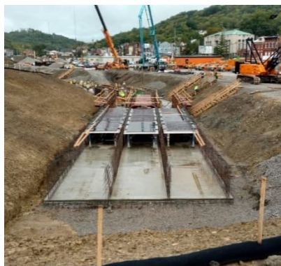
Three-cell, box conduit during construction. The top of the box conduit serves as the bottom of the urban waterway channel.
