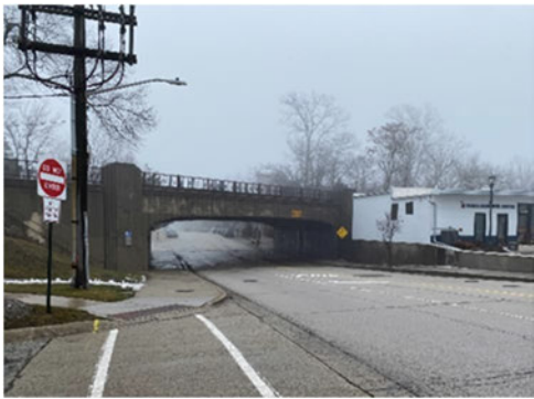
Winnetka Avenue underpass.
