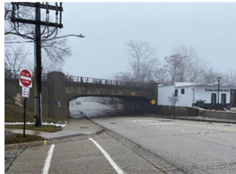
Winnetka Avenue underpass.
