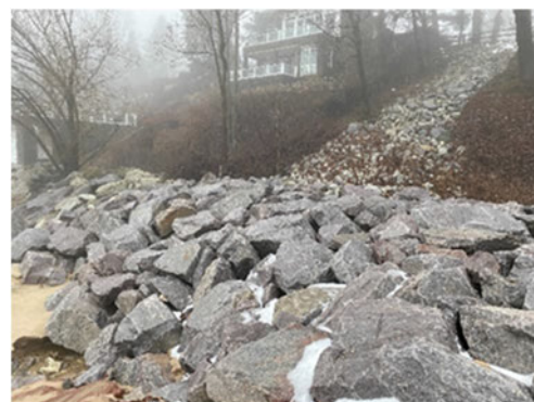
Lloyd Park/Boat Launch outfall.
