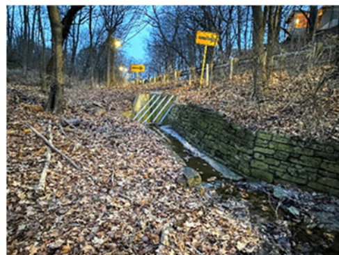
Ravine from Old Green Bay Road and the culvert under Sheridan Road.
