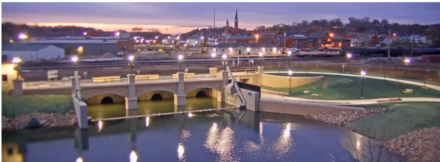
Post-Construction photo of the outfall, level control gate, and pedestrian tunnel at the CPR crossing.
