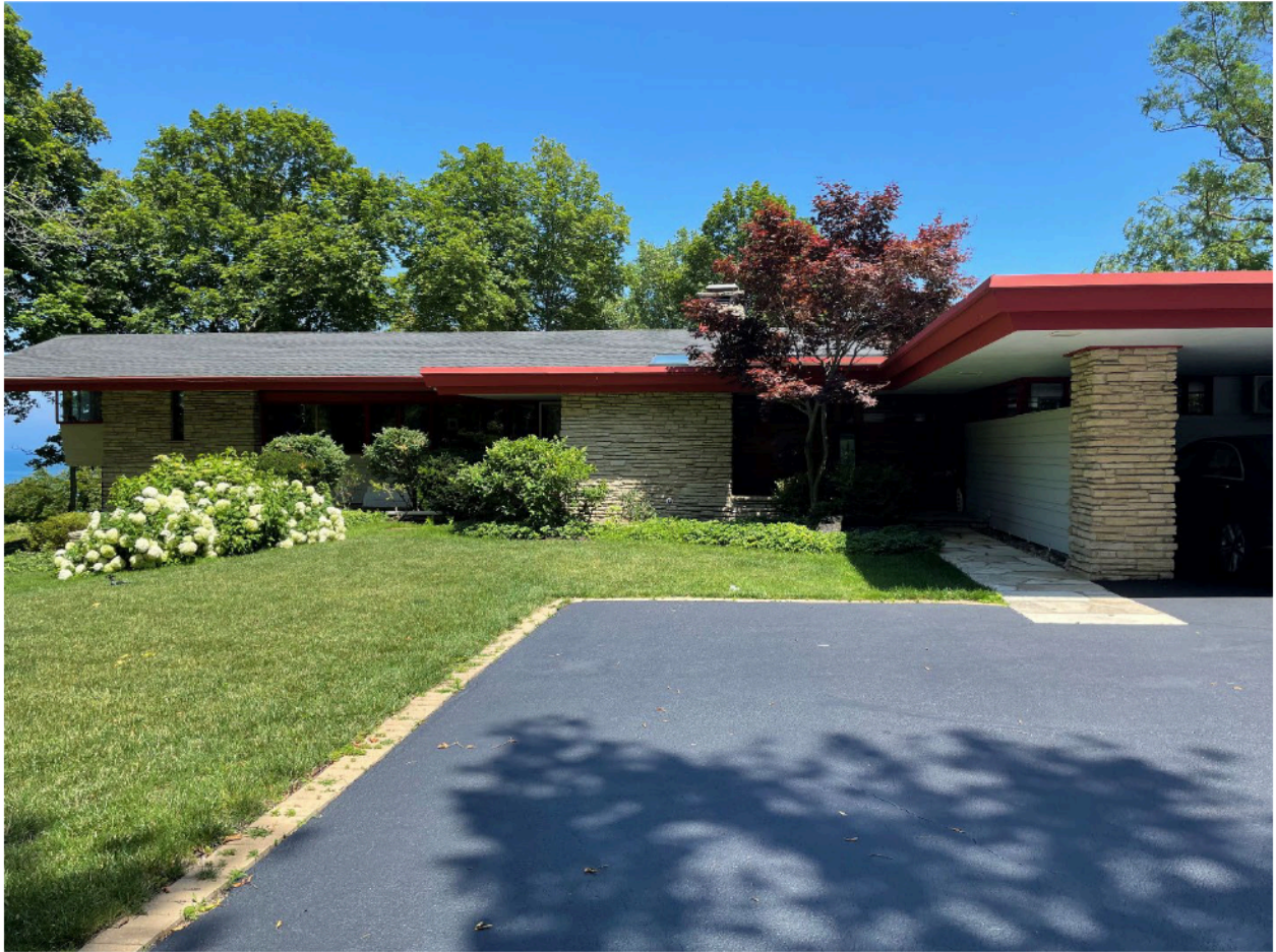
Figure 3 Front elevation of the Arno and Verna Myers House.
