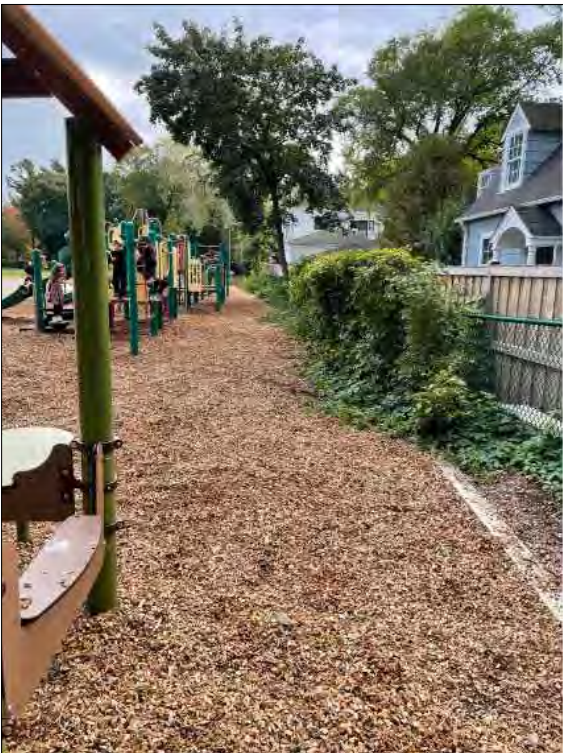
SITE PHOTOS SITE CONDITIONS
