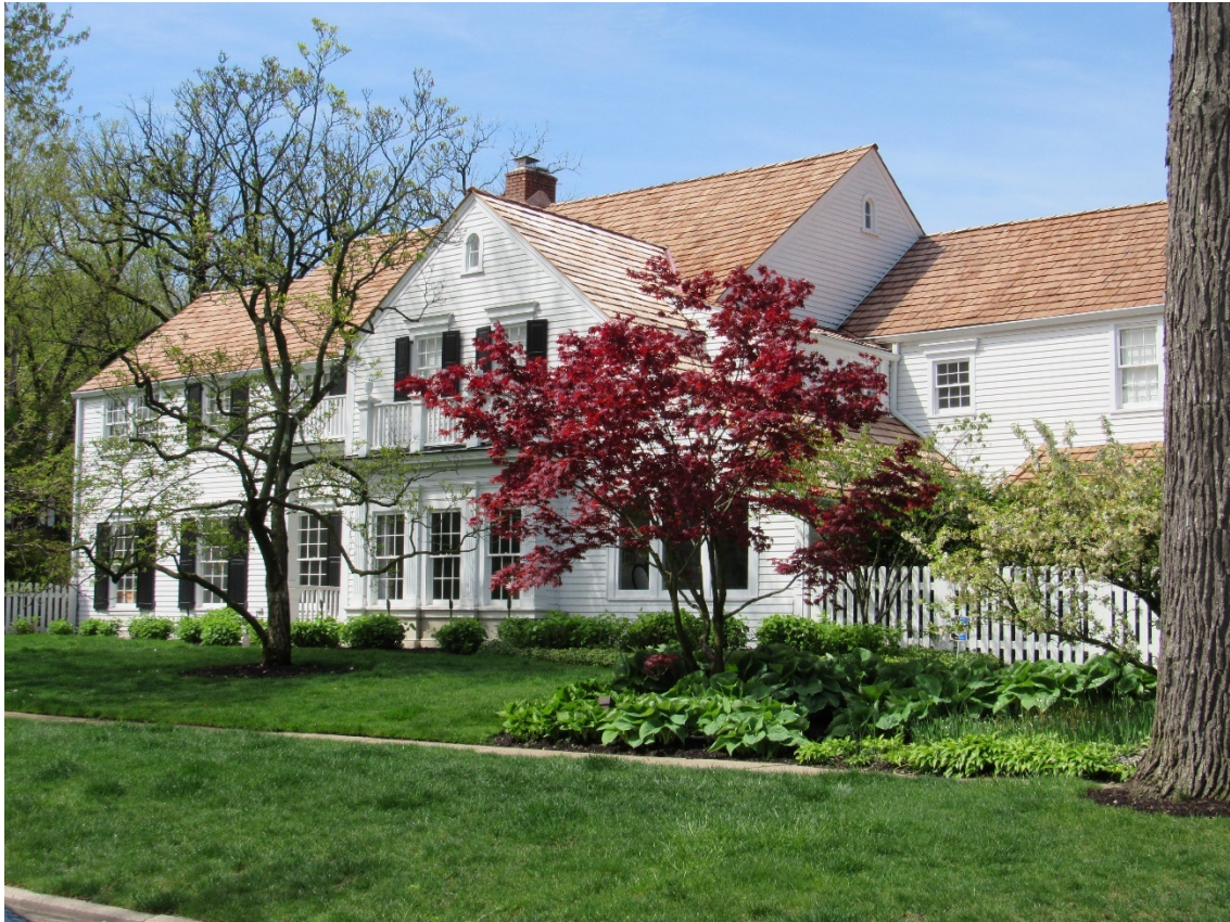
Figure 4 – Subject Property - Partial East and North Elevations
