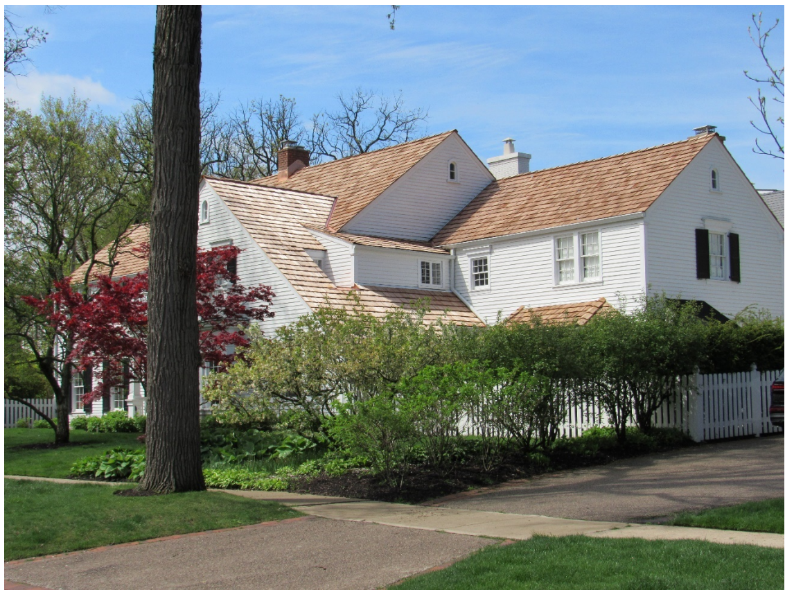
Figure 5 – Subject Property – North (Rear) Elevation
