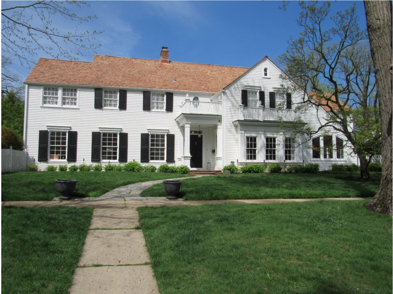
Figure 3 – Subject Property - Corner Elevation (Locust Street)
