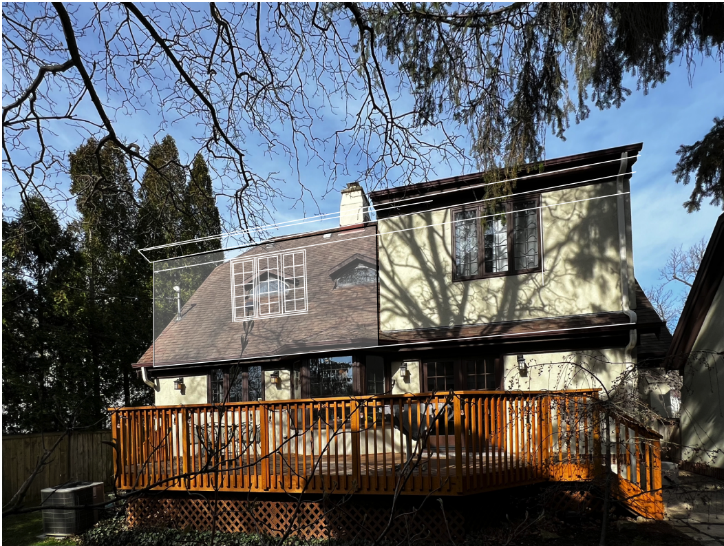
4 SIDE OF HOME LOOKING EAST W/ ADDITION
